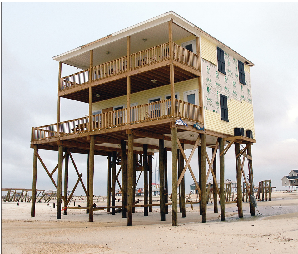
Figure 3-11. Example of well-elevated and embedded pile foundation tested by Hurricane Katrina. Note adjacent building failures (Dauphin Island, AL, 2005).
