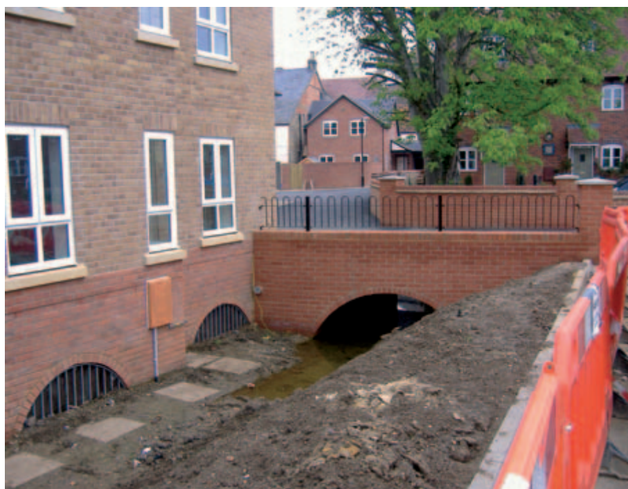
Figure 5.3 Flood management system (courtesy of Leadbitter Construction)
