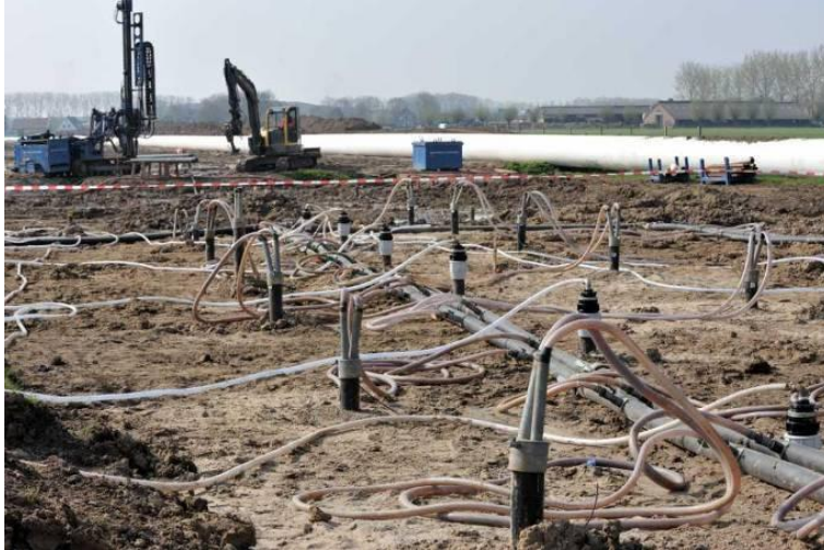
Figure 5.2 Cementing gravel for the horizontal drilling pilot near Nijmegen, 2010
