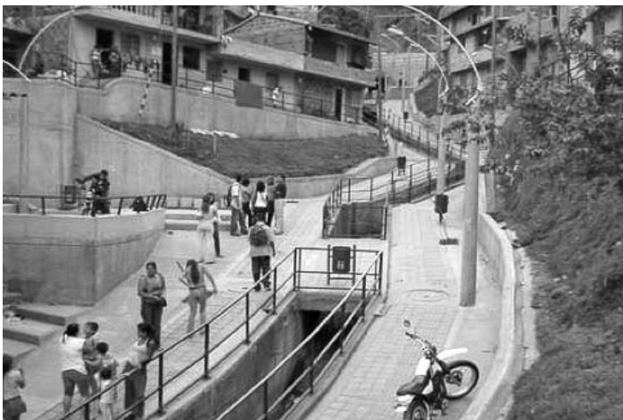
Photo 3.6: Reconstructed urban drainage in Acapulco, Source: UN-HABITAT
