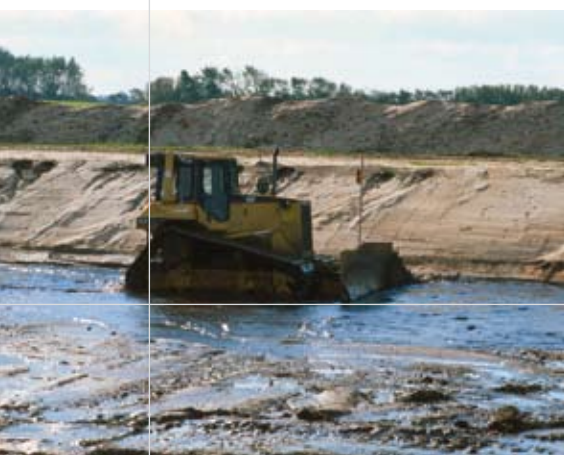
Reconstruction work on the River Skjern
