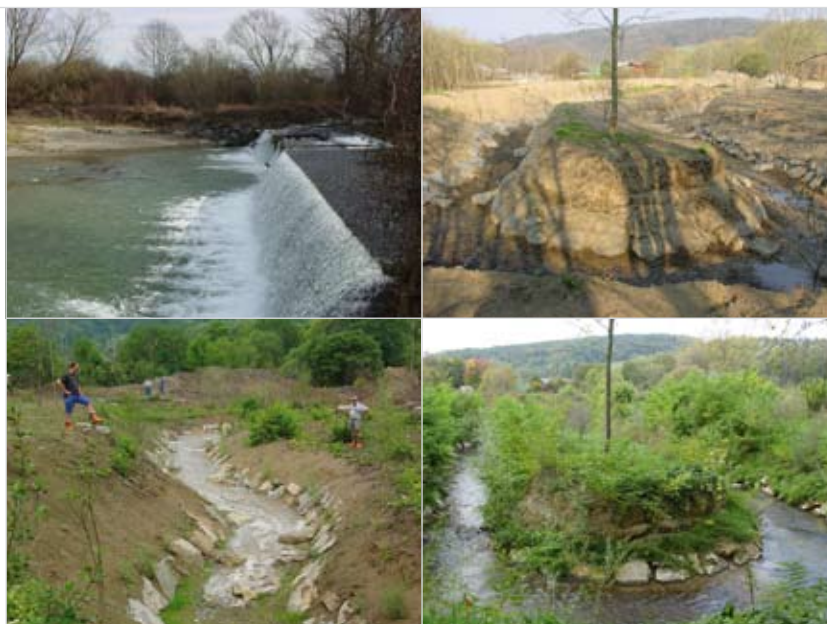
LIFE project work – top (left to right): opening a new side channel that allows for the migration for fish at the weir 'Eibelsau' – weir, and construction of the side channel – below (left to right) first water flowing into the new channel, and channel with flowing water and vegetation allowing the fish to migrate upstream
