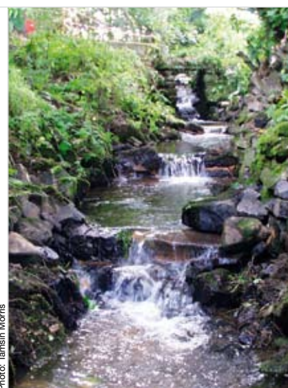
A stepped fish pass installed to allow migrating fish access to upstream spawning grounds
