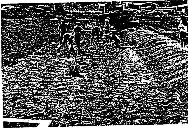
13. After flooding the wetland to settle the substrate, the wetland should be drained for planting.
