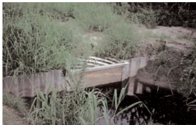
Figure 13-15 Pipe drop inlet structure
