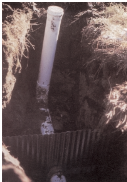
Figure 13-17 PVC riser being installed at broken tile will raise water level.
