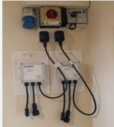
**Figure 1** Sump pump controls are on separate circuit, fixed high above water level
