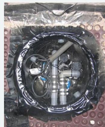
**Figure 4** Two sumps (similar in size to a domestic dustbin) contain pumps designed to operate at different water depths.
