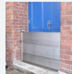
**Figure 1** Demountable barrier for external door 1 donated by [www.floodtec.co.uk](http://www.floodtec.co.uk)
