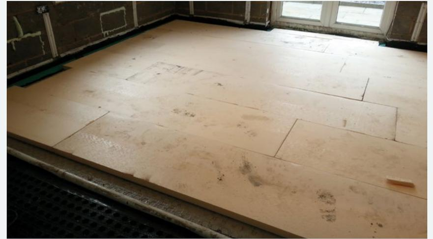
**Figure 6** Closed cell (waterproof) insulation on the floor
