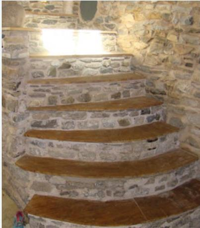
**Figure 6** Resilient (& very attractive) steps to upstairs flat (replaced standard wooden staircase)
