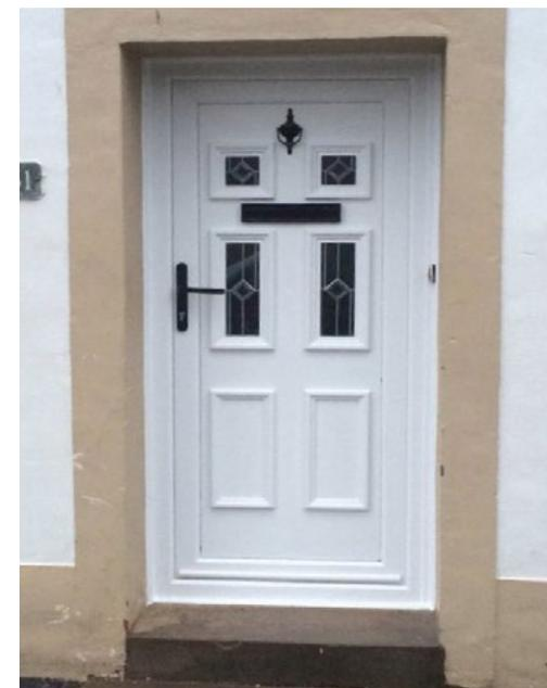
**Figure 5** A flood-resistant door has been installed, which allows additional time for moving items before the water has to be let in. Installation by Floodsafe Projects Ltd ([www.floodsafeprojects.co.uk](http://www.floodsafeprojects.co.uk))
