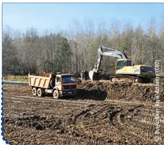
Works to improve the river lateral connectivity and dynamics: earth embankments removal
