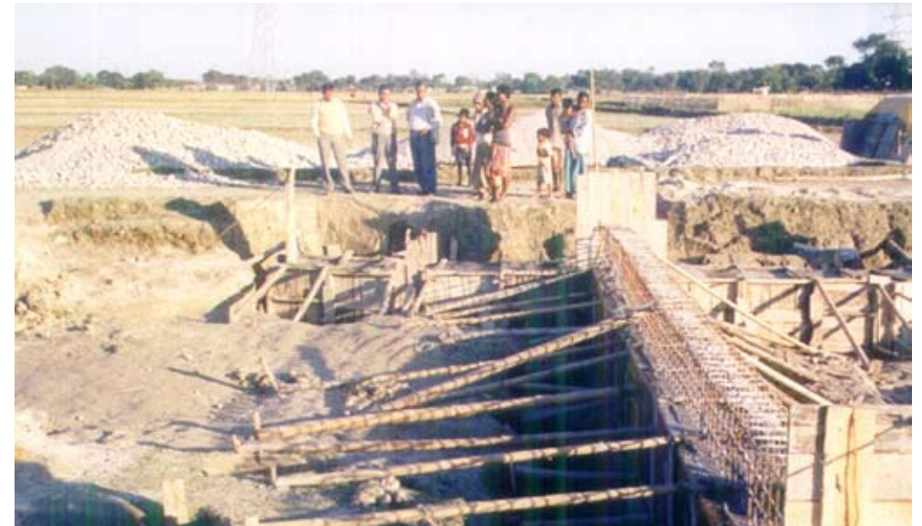
Figure 2: Constructing a gully plug to retain groundwater
