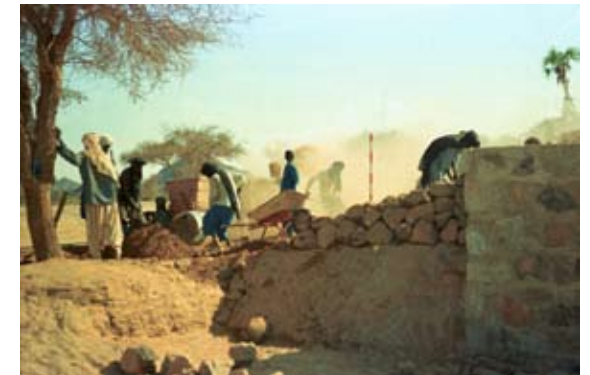
Figure 2: Construction of diversion works
