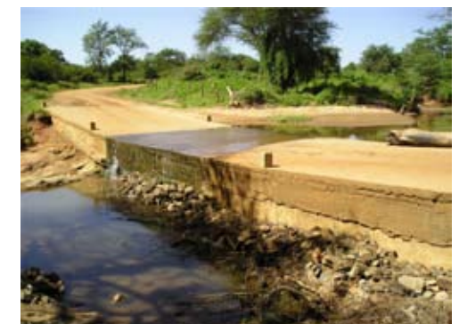
Figure 3: Irish bridge (Source: Nissen-Petersen, E, 2006)
