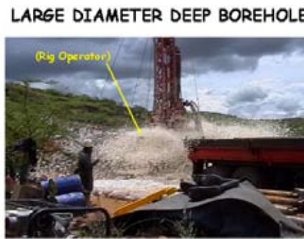
Figure 4: Drilling of large diameter deep borehole
