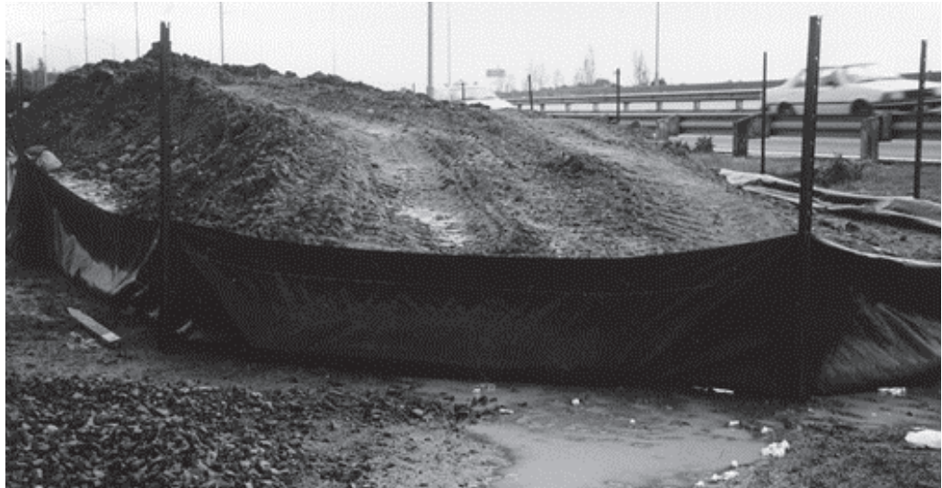
Figure 6.13 A silt fence around a stockpile.
