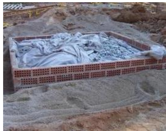
Figure 2.24. Construction of a soakaway in Barcelona (Spain).
