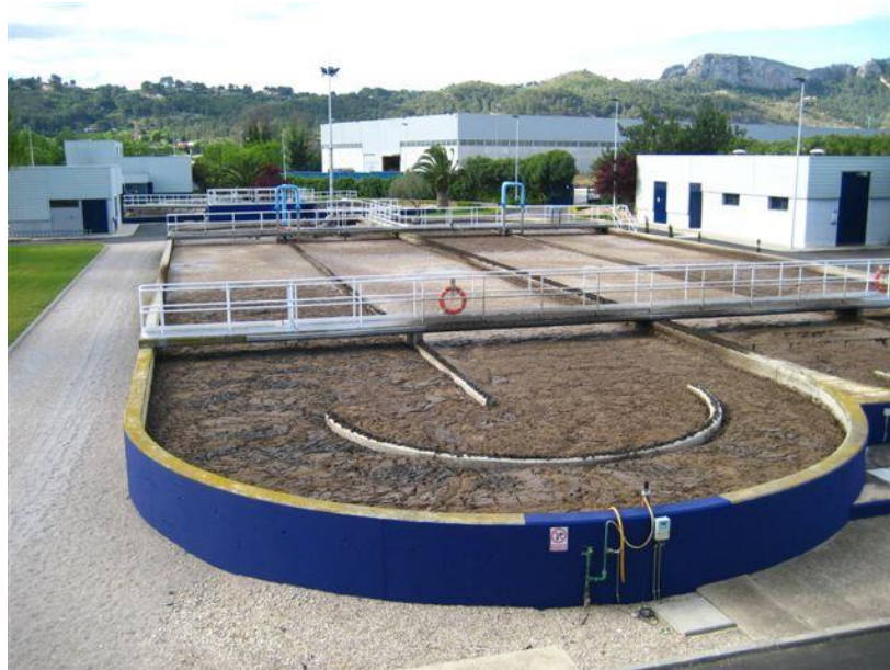
Figure 2.13. Wastewater treatment plant in Xàtiva (Spain).
