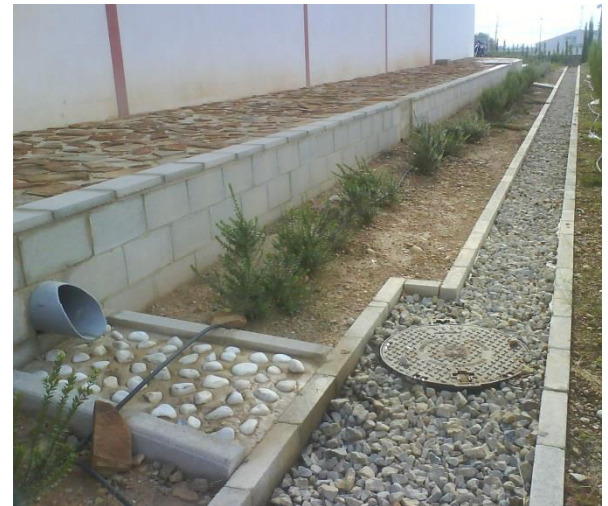
Figure 2.36. Filter drain in Crevillent, Spain.
