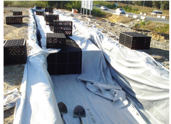
Figure 2.28. Construction of a geocellular system in Oleiros, Spain.
