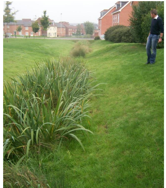
Figure 2.38. Vegetated swale in Leicester (England).
