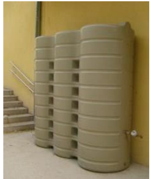
Figure 2.18. Water butts in Xàtiva (Spain).
