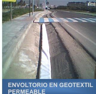
ENVOLTORIO EN GEOTEXTIL PERMEABLE
