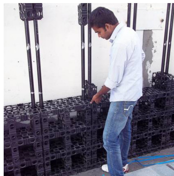
An installer assembling a Gro-Wall® PRO
