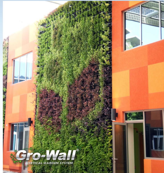
U.A.E, an installation of 220m 2 of Green Wall into a school project. The Green Walls lower ambient temperature in the hot desert environment.
