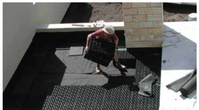
Installing Flo-Tank® modules into planter box.
