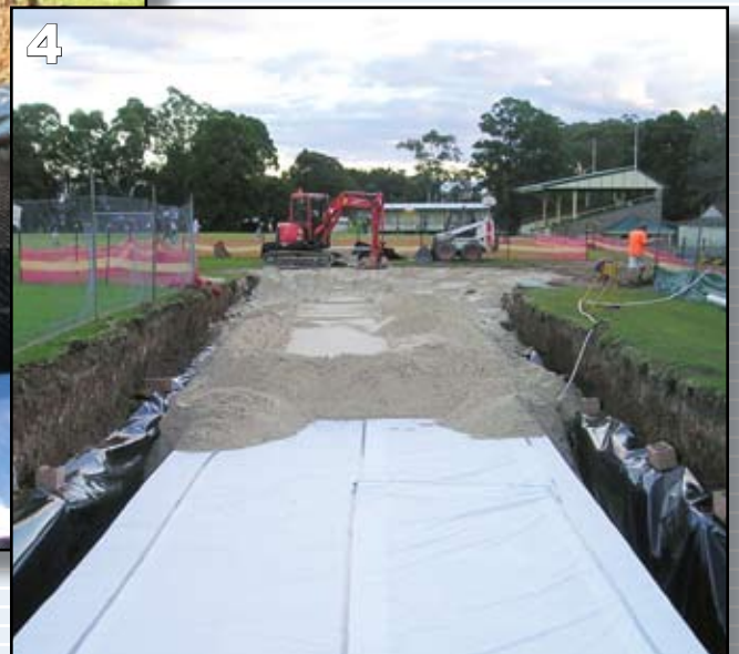
Backfilling with washed river sand.
