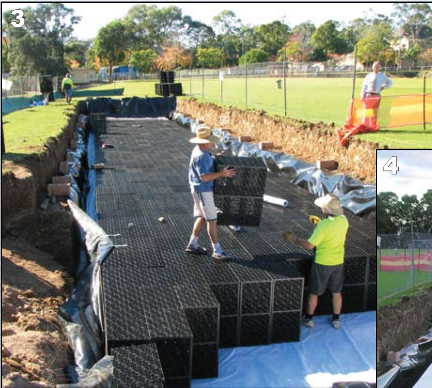
Installing Flo-Tank® modules.
