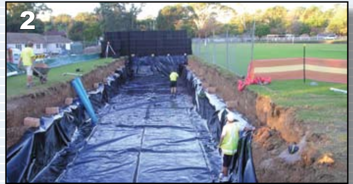
Installing Liner for Water Retention.
