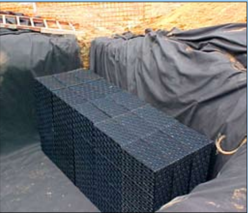
Installation of Matrix® tank modules for infiltration tank application.
