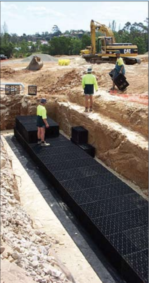
Installation of Infiltration Tank.
