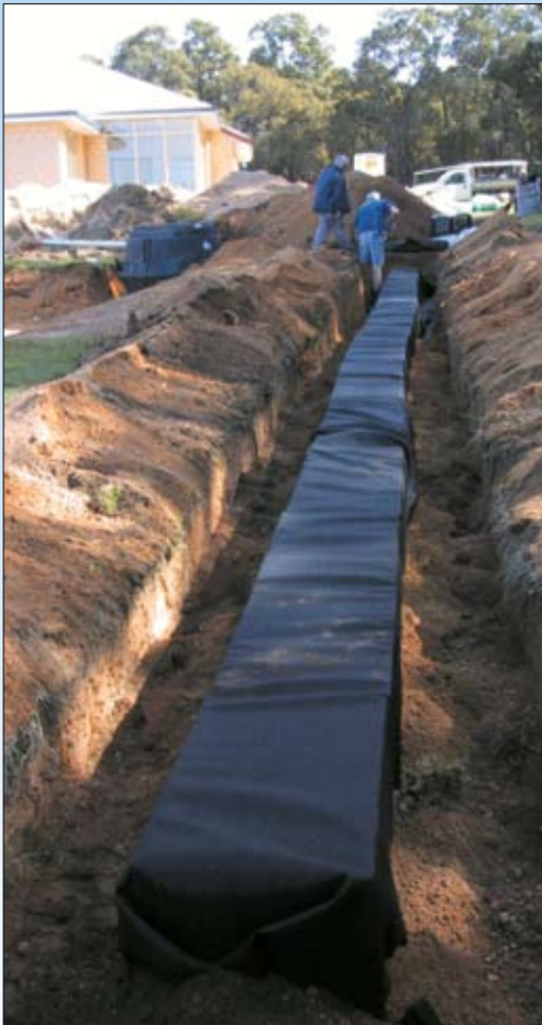
Installation of Leach Drain System.
