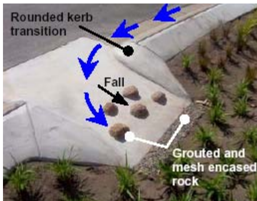
Figure 10.12 Kerb Inlet Concept Diagram
