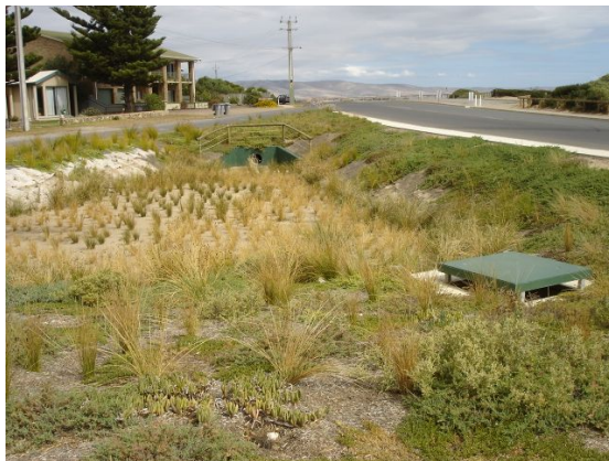
Figure 1.3 Bioretention Basin, Palmer Road, Aldinga Beach
