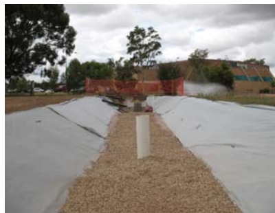
Figure 10.13 Preliminary Stages of Construction of a Bioretention Swale at Mawson Lakes Campus at the University of South Australia
