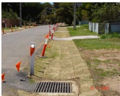
Figure 2.3 Retrofit of Street with a Swale, City of Onkaparinga
