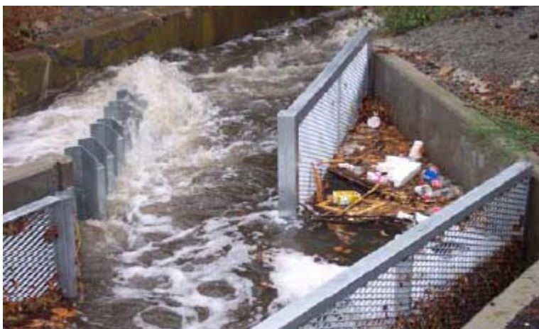
Figure 9.9 Vane Style Diversion Weir, Sebastopol, Victoria
