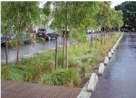
Figure 10.9 Kerb Inlet Design for a Bioretention Swale
