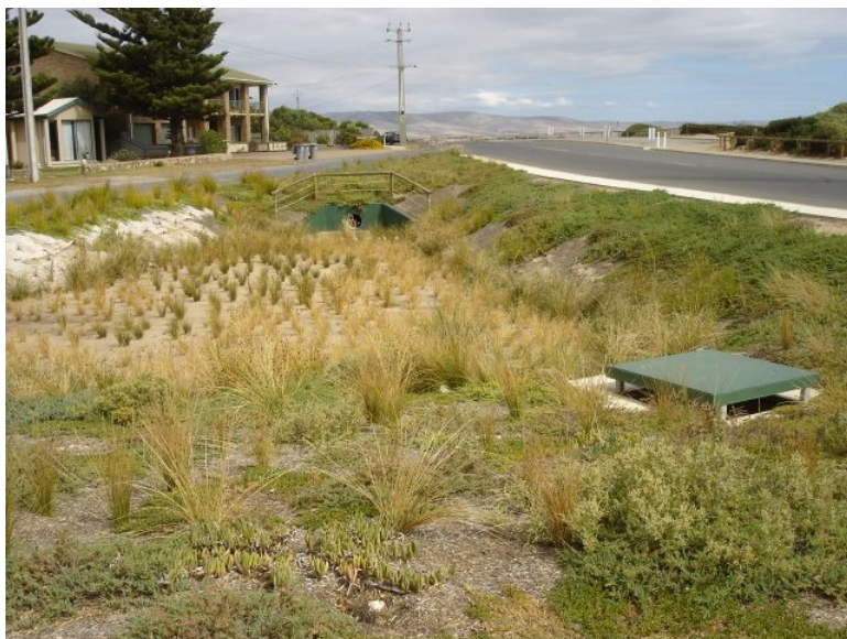
Figure 10.7 Bioretention Basin at Palmer Street, Aldinga Beach
