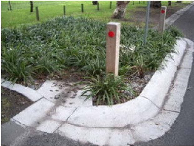
Figure 10.10 Kerb Inlets Design for Bioretention Basin
