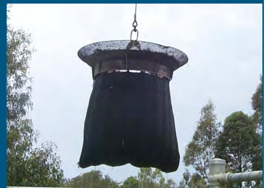
In-Ground GPT Basket Being Removed for Cleaning
