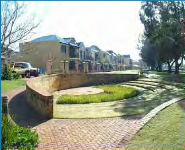
Ascot Waters stormwater detention basin
