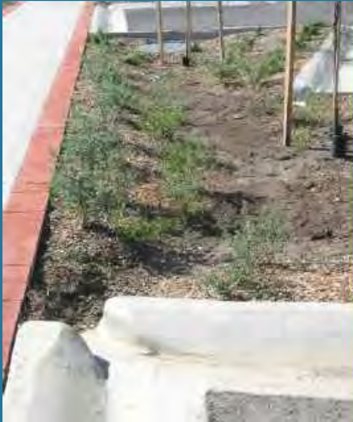
Interrupted kerbs direct stormwater to treatment facilities
