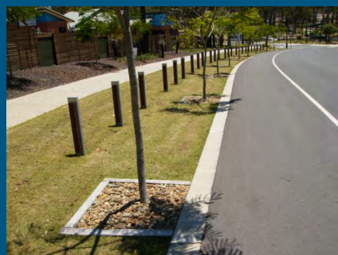
Kerb without Set-Down, showing sediment accumulation on road.
