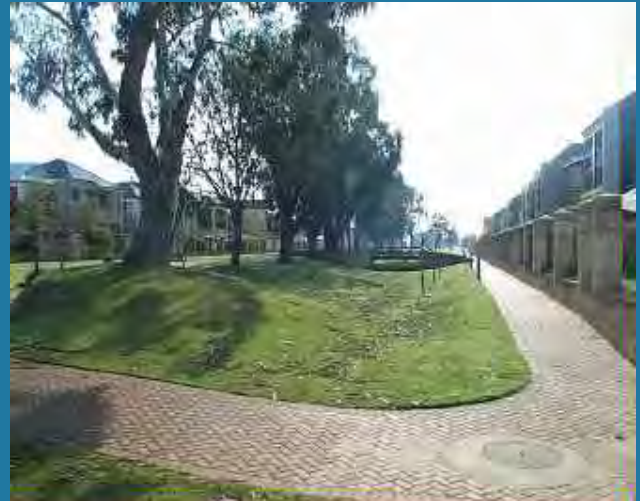
A vegetated swale drain at Ascot Waters
