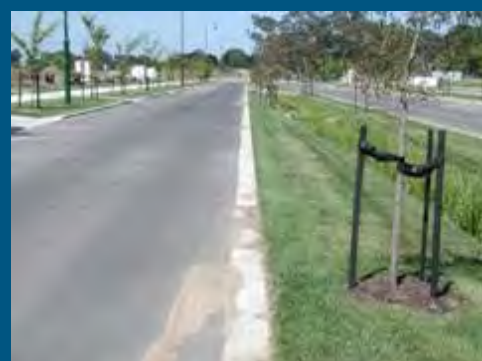
Kerb without Set-Down, showing sediment accumulation on road.
