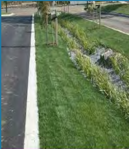
Lynbrook Estate bioretention system
