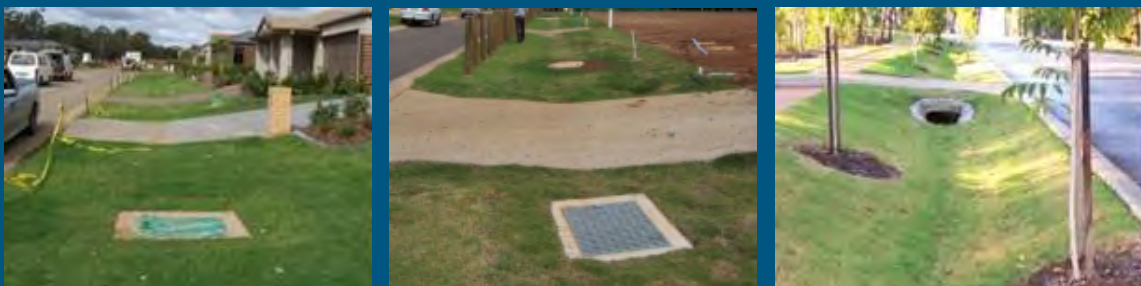
Driveway Crossings: At-grade (left) under construction with trees yet to be established, pre-constructed 'at-grade' (centre) and elevated driveway crossings to allow vehicle access across swales
