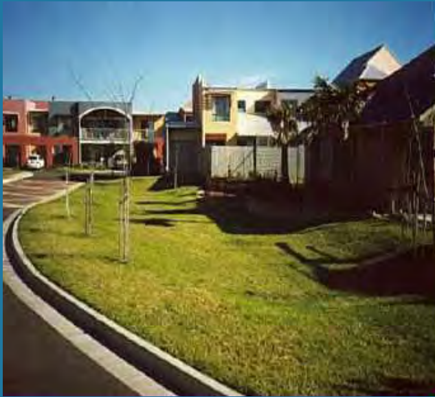
Figtree Place detention basin under dry and wet conditions
