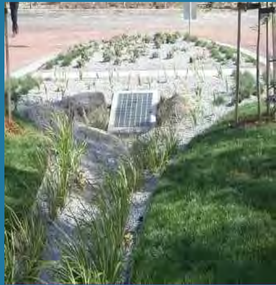
Overflow pit at the base of a bioretention system
