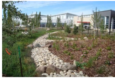
Bioswale at Terwillegar Recreation Centre, Edmonton, AB to treat roof runoff. Photo by Xiangfei Li, City of Edmonton.
