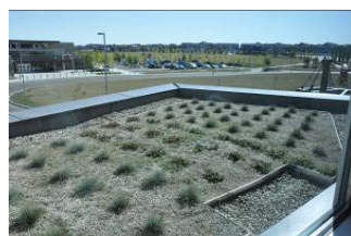
Newly planted green roof at Terwillegar Recreation Centre showing perimeter drainage, Edmonton, AB. Photo by Xiangfei Li, City of Edmonton, 2011.
