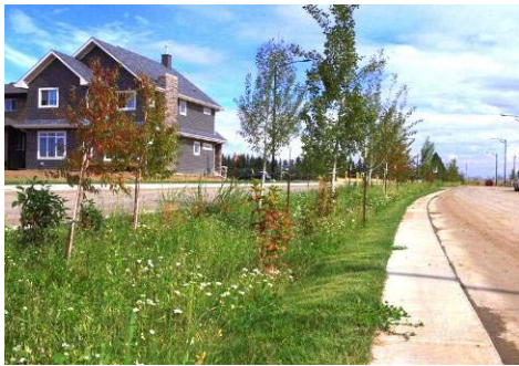
Bioswale at Big Lake Trumpeter neighbourhood in Edmonton, AB to treat roadway runoff. Photo by Xiangfei Li, City of Edmonton.
