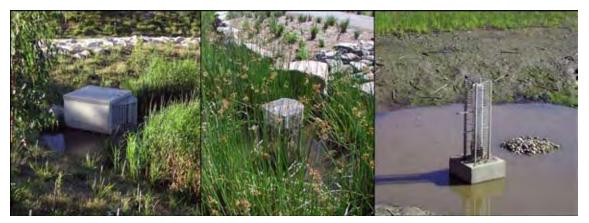
Figure 6. Debris guard examples for riser outlets. (Source: Morton Bay Waterways & Catchments Partnership 2006.)
