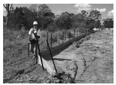
Figure 5. Silt fence for controlling sediment during land development. (Photograph: André Taylor, Ecological Engineering Pty Ltd.)
