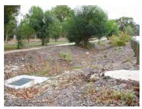
Figure 7. Bubble-up pit located within a swale at the downstream end of the catchment. (Photograph: Department of Water 2007.)
