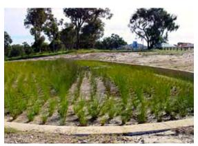
Figure 2. Bioretention area constructed in the Treendale development, Australind. (Photograph: Wayne Edgeloe, Thompson McRobert Edgeloe (TME) Consultants, 2006.)
