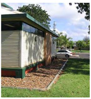
Pervious surface under gutterless roof, Shire of Broome. (Photograph: Allan Ralph, Shire of Broome 2005.)
