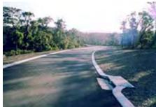
Figure 7. Central drainage linked to soakwells and detention area. (Source: TME 2003.)
