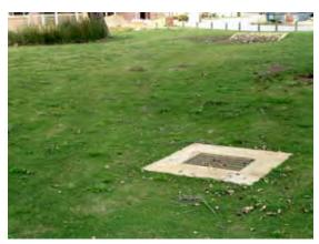
Figure 5. Grassed swale and bubble-up. (Photograph: Department of Water 2006.)
