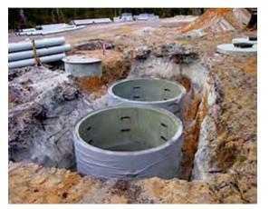
*Figure 5. Soakwell construction. (Photograph: TME 2003.)*
