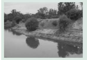
Figure 1. Sediment excavated from the Harvey Main Drain and stockpiled on the banks. Sediment has buried fringing vegetation and may be washed into the waterway. (Photograph: Department of Environment.)
