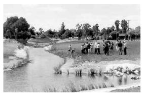
Figure 24b. Bannister Creek post-engineering (restoration) works summer 2001. The channel was realigned to create a winding creek and the banks reshaped to a gentle slope and stabilised. (Photograph: Department of Environment.)
