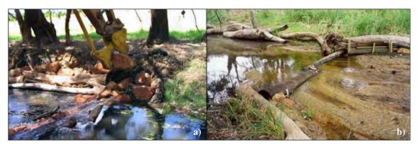
Figure 5. a) Construction of a log and rock riffle structure in the Canning River, Pioneer Park, Gosnells. (Photograph: Department of Water 2004.) b) Log riffle built on the South Dandalup River, Pinjarra, to stabilise the sandy riverbed, induce a scour pool and enhance habitat diversity. (Photograph: Water and Rivers Commission 1999.)
