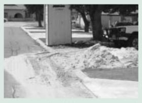
Figure 5. Sand stockpile erosion onto a road. (Photograph: Clean Site, Keep Australia Beautiful Council WA.)
