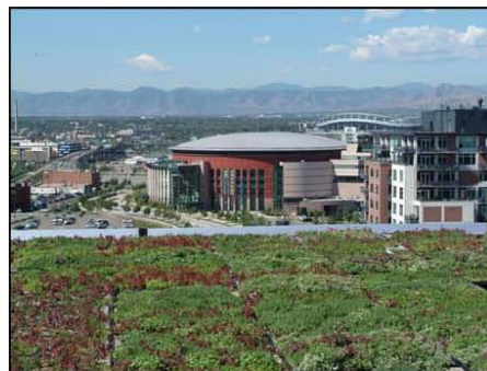
Green roofs capture rainfall, promote evapotranspiration, and offer energy savings. This is a photo of a green roof on the EPA Region 8 building in Denver, CO.
