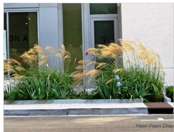
A curb cut and bioswale at 1100 S. Hope Street in downtown Los Angeles.
