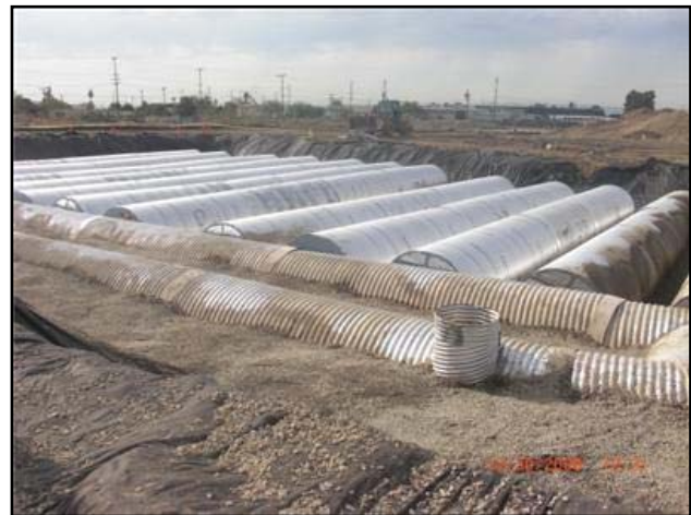
Underground Infiltration Units Lowe's, Pacoima
