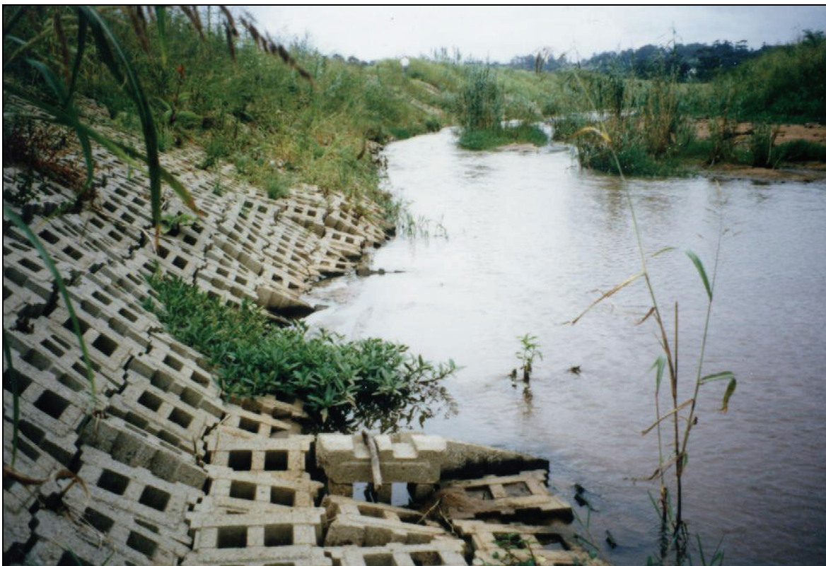
Photograph 5.6: Flexible concrete mattress failure due to weak supporting soils
