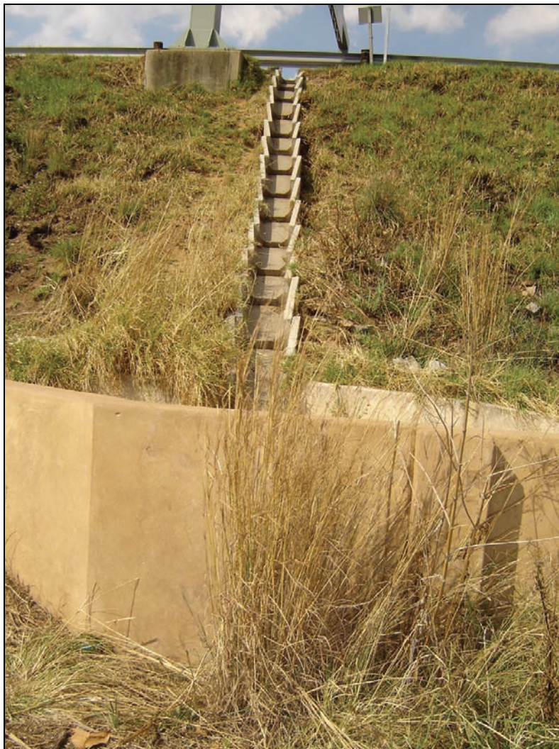
Photograph 5.11: Discharge chute, prefabricated blocks
