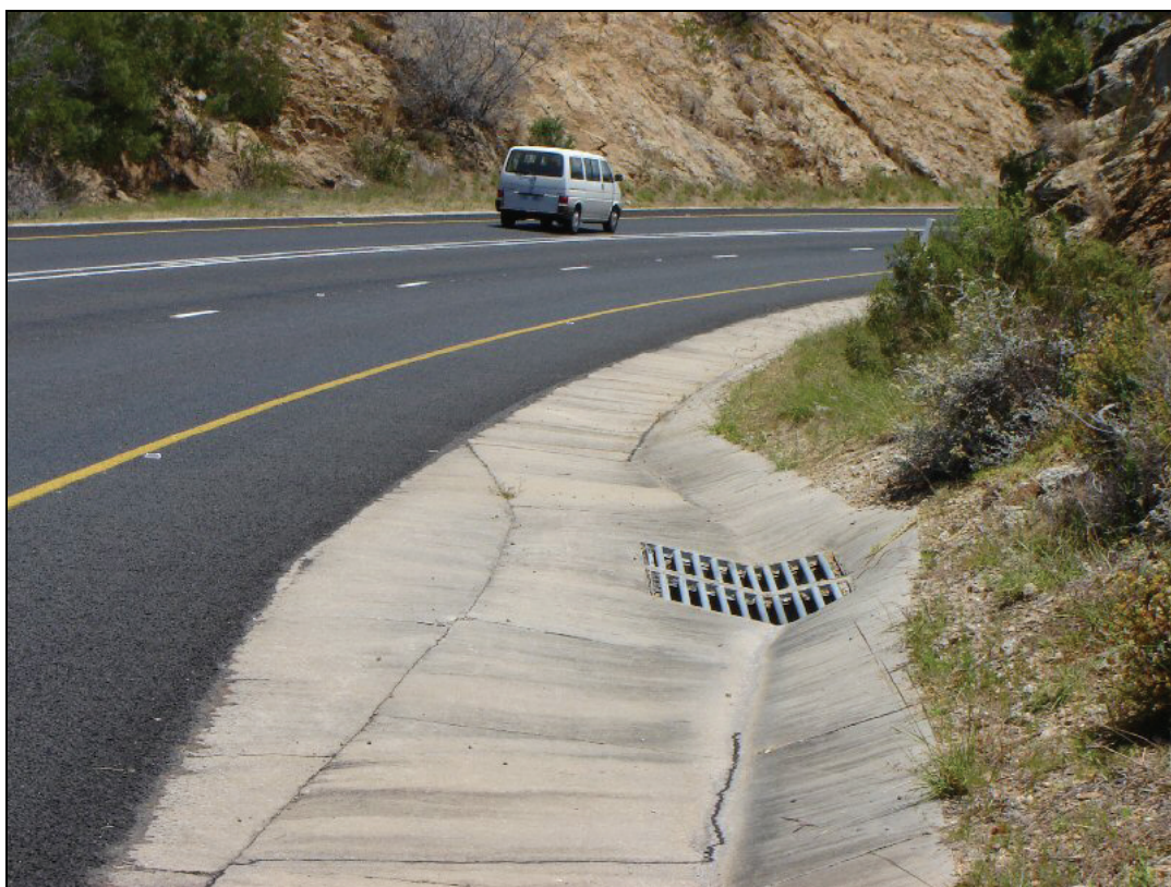
Photograph 5.3: Concrete side drain with grid inlet
