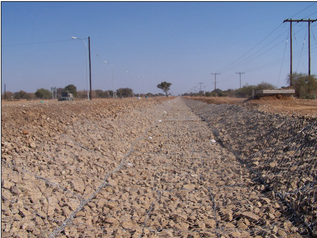
Photograph 5.8: Gabions used for erosion protection (Courtesy: Land Rehabilitation Systems)
