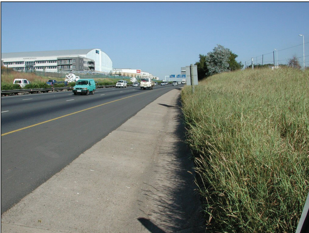
Photograph 4.5: Concrete side drain. Estimated roughness = 0,002 m (Manning n-value = 0,016 s/m 1/3 )
