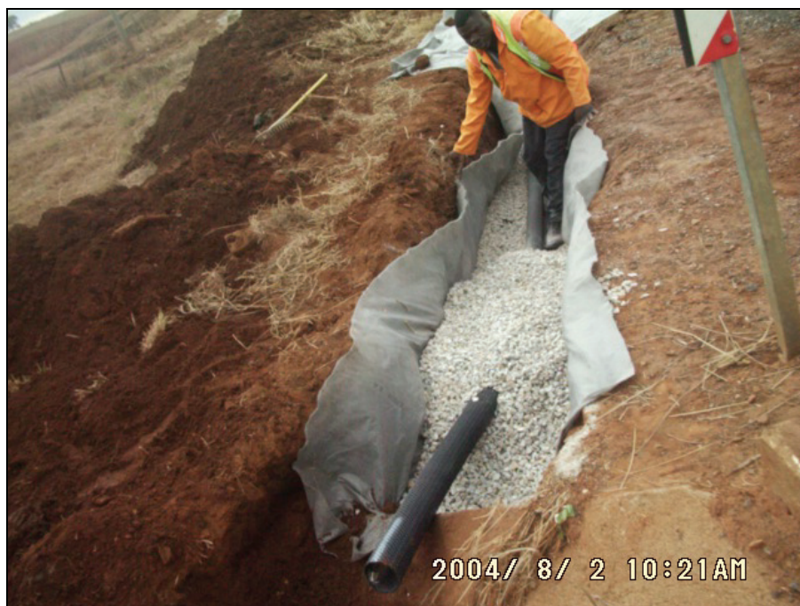
Photograph 9.2: Installation of sub-surface drainage to improve the drainage
