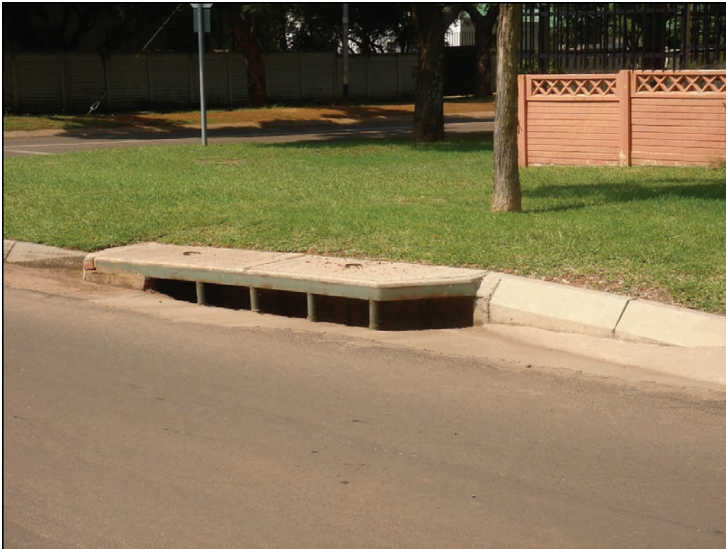
Photograph 5.1: Detail of a typical kerb inlet with a transition (side outlet)
