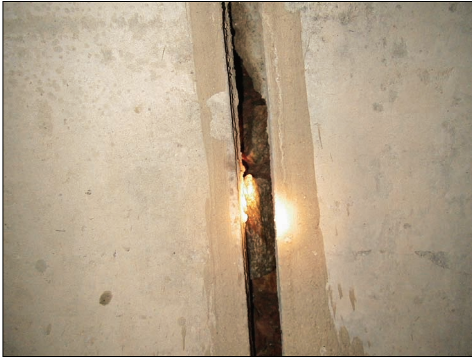
Photograph 7.1: Piping (flow path through culvert joint eroding dispersive material) (Courtesy of: MVD Consulting Engineers)
