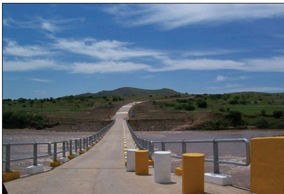
Photograph 6.4: A low-level crossing on Tsitsa River with provision for pedestrians
