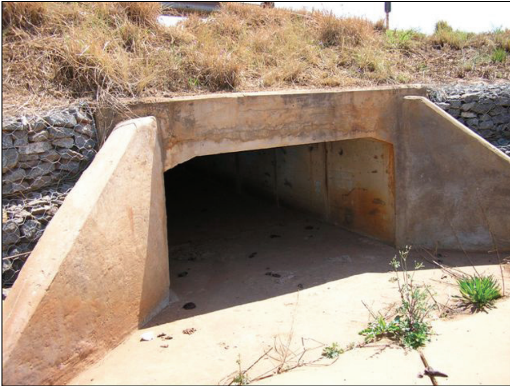
Photograph 7.2: Typical culvert with wingwalls
