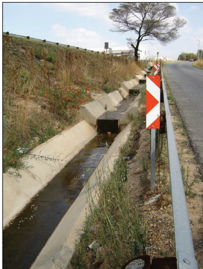
Photograph 5.10: Stepped energy dissipator along the N3
