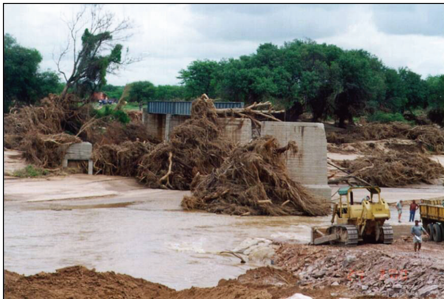
Photograph 8.1: Failure partly due to debris build-up
