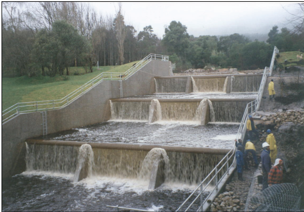
Photograph 5.9: Stepped energy dissipator (Hout Bay River, Cape Town)
