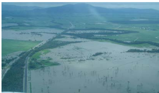
Figure 3.2.2 – Murray River Crossing of Bruce Highway
