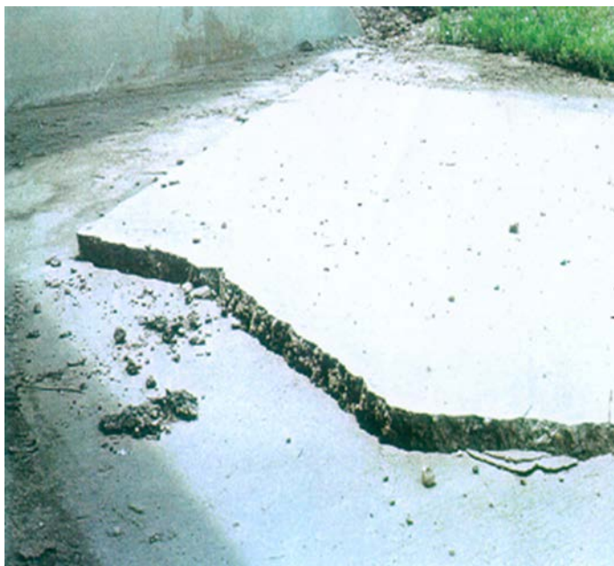
Figure 9.2.7(b) – Vertical displacement of apron failure
