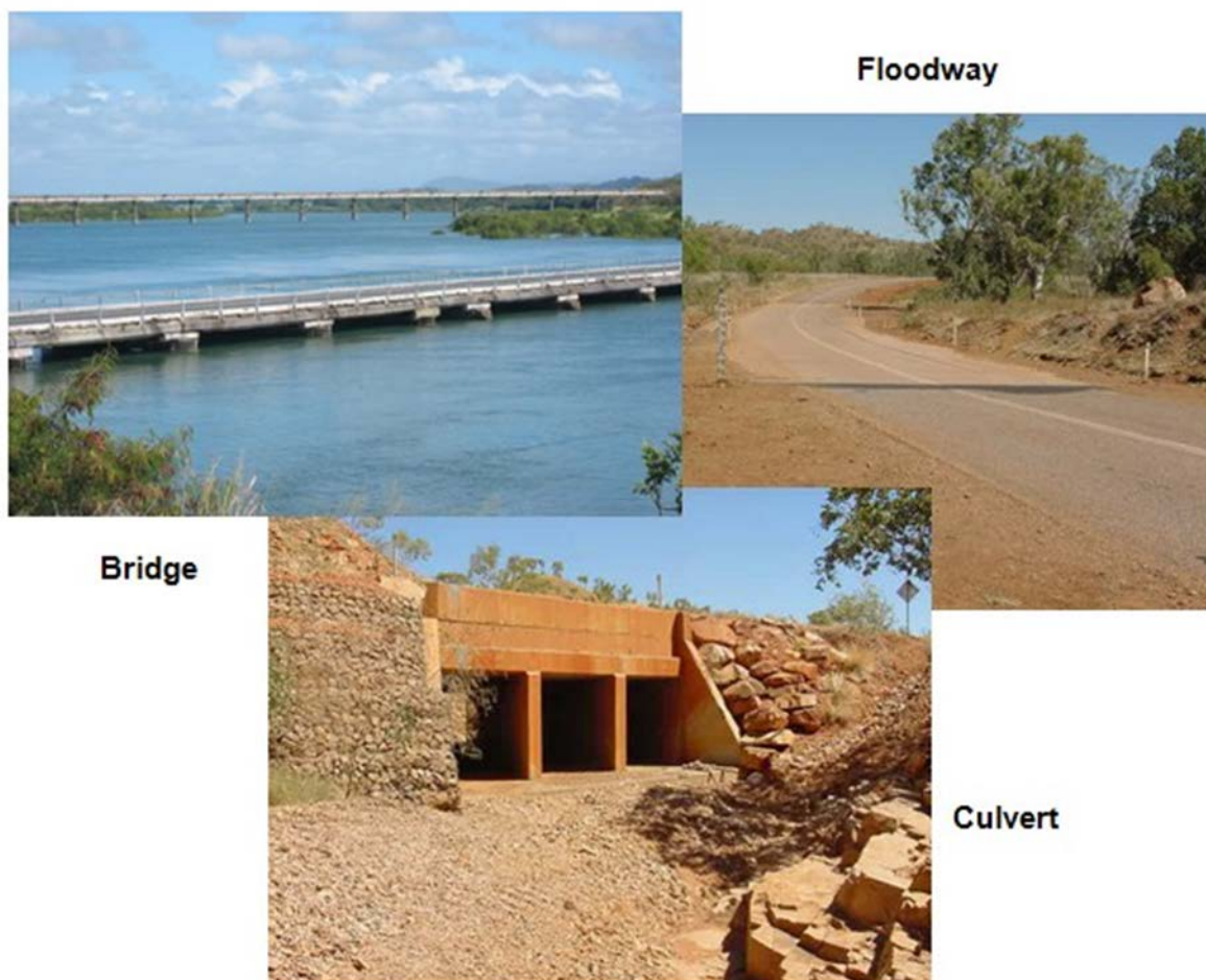
Figure 2.3.5.1 – Primary drainage infrastructure types
