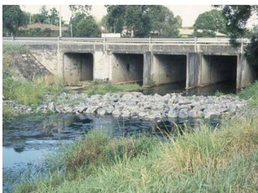
Figure 9.5 – Box culverts with riprap
