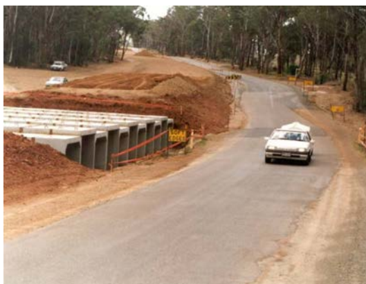
Figure 9.2.6.6 – Slab link box culvert under construction
