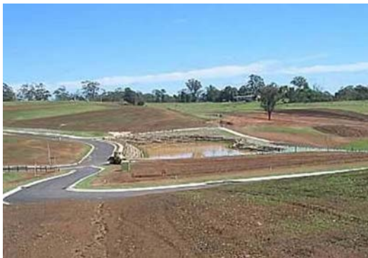
Figure 3.3.3 – Detention basin in a residential subdivision
