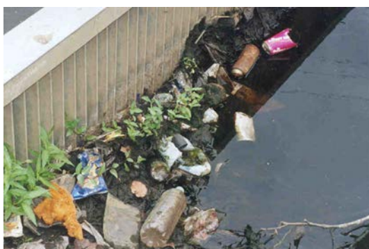
Figure 7.5.3.1(b) – Trash rack and pollutants
