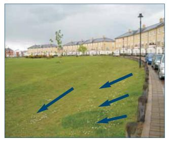
Figure 1.3 Runoff flowing into a swale as part of public open space, Ipswich, England
