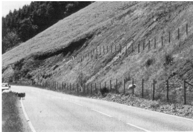
Plate 2D Trial of vegetative slope stabilisation on a highway cutting. Experimental panels in the foreground, with a typical untreated slope in the background. Sheep have been introduced into the lower half of the trial to assess the effect of grazing
