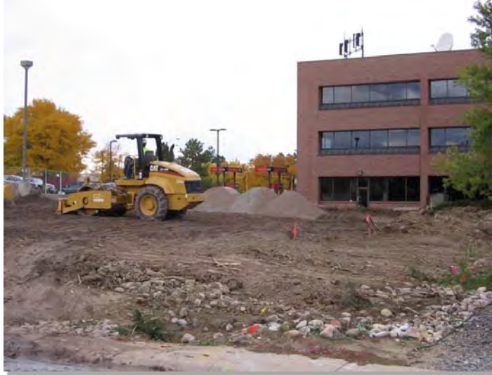
Photograph B-5. Rain garden is staked out at the low point of the parking area prior to excavation.
