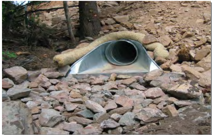
Photograph TOP-1. Riprap outlet protection.
