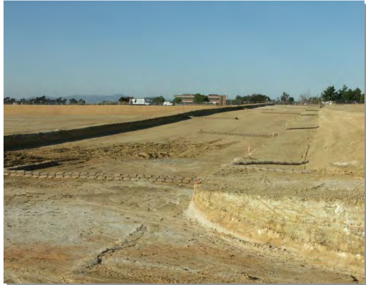
Photograph RCS-1. Rough cut street controls.
