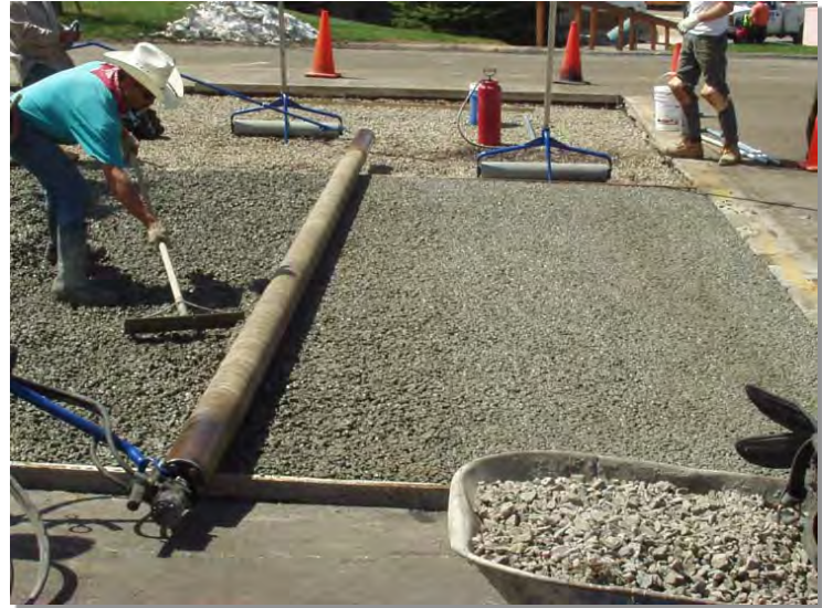
Photograph PC-1. Construction of pervious concrete at the UDFCD stormwater monitoring site in Lakewood, CO, in 2004.
