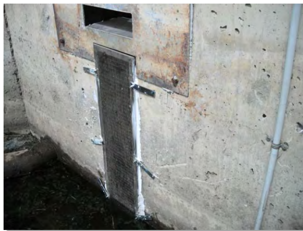
Photograph OS-3. Trash rack after repair.
