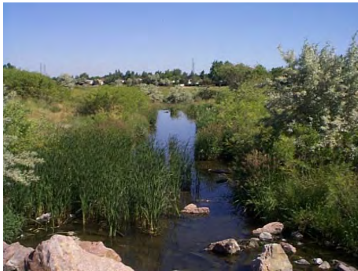
Photograph CWC-1: Constructed wetland channels treat stormwater through straining, settling, and biological processes.
