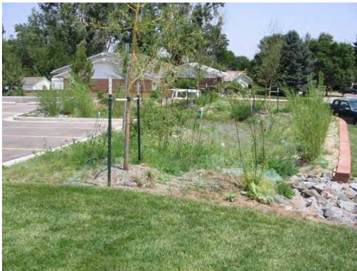
Photograph B-8. Shrubs and trees are placed outside of the ponding area and away from geotextiles.
