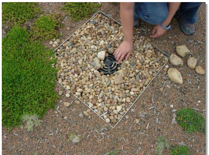
Photograph GR-3. Metal edging separates growing media from rock that surrounds the roof drain. It also serves to facilitate regular maintenance by limiting plant and root growth near the drain.
