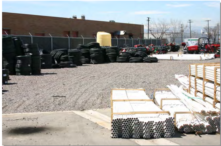
Photograph PG-1. This Denver installation of porous gravel provides volumetric treatment of the WQCV as well as a material storage area.
