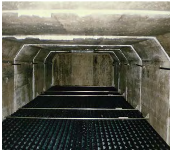
Photograph UG-2. Maintenance access to all chambers of an underground BMP is an important design consideration. Photo courtesy of Robert Pitt.
