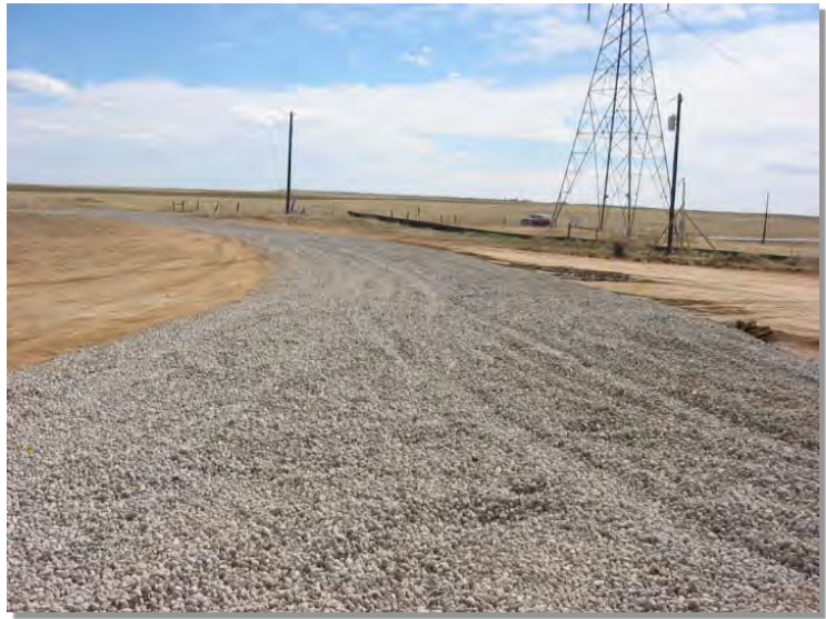
Photograph SCR-1. Stabilized construction roadway.
