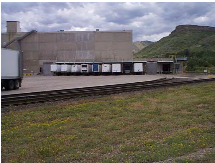
Photograph CS-1. Covered truck loading dock helps reduce exposure of materials to runoff.
