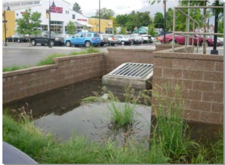
Photograph EDB-3. Although walls may complicate maintenance access, this outlet structure is relatively hidden from public view. This photo was taken shortly following a storm event.
