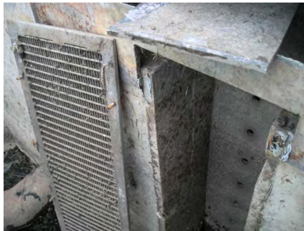
Photograph OS-2. This trash rack could not be properly attached due to its inadequate flange width.
