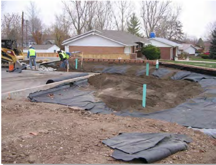
Photograph B-7. The aggregate layer is covered with a geotextile and growing media. This photo shows installation of the geotextile to separate the growing media from the aggregate layer below. Cleanouts for the underdrain system are also shown. Note: The current design section does not require this geotextile.
