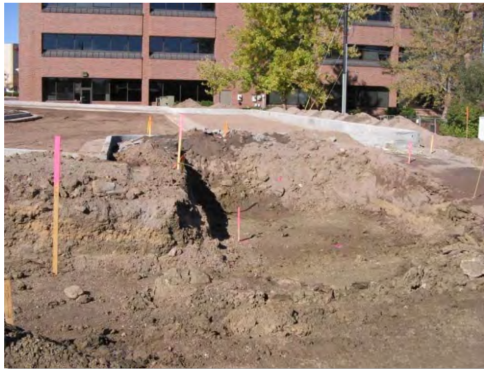
Photograph B-6. Curb and gutter is installed. Flush curbs with wheel stops or a slotted curb could have been used in lieu of the solid raised curb with concentrated inflow.
