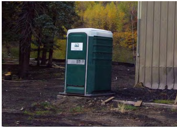
Photograph GH-3. Locate portable toilet facilities on level surfaces away from waterways and storm drains. Photo courtesy of WWE.
