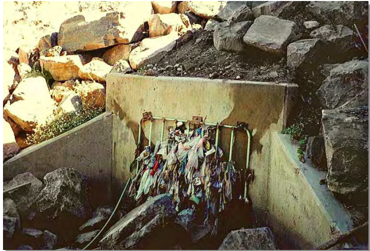
Photograph SSC-1. Storm drain cleaning may help to remove pollutant sources and helps to maintain the capacity of the storm pipes.
