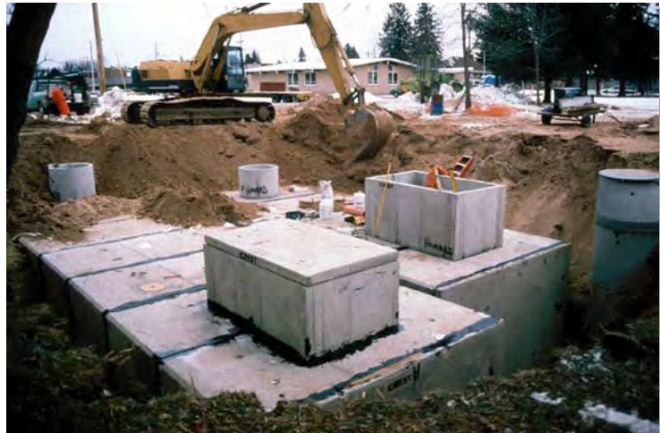
Photograph UG-1. Installation of an underground BMP (Photo courtesy of Robert Pitt).
