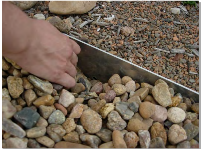
Photograph GR-2. The metal edge shown in Photo GR-2 has perforations near the bottom to allow flow into the drain.
