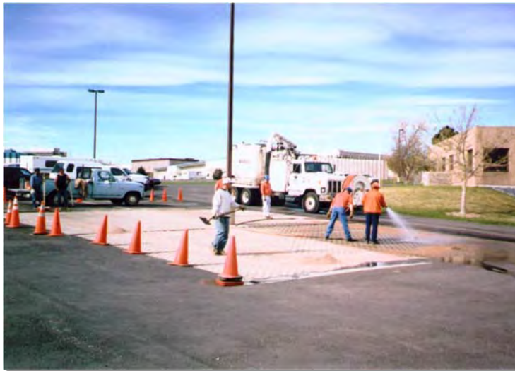
Photograph CGP-2. The Lakewood concrete grid pavement installation was one the first permeable pavement stormwater monitoring sites constructed by UDFCD. This photo was taken following construction in 1994.
