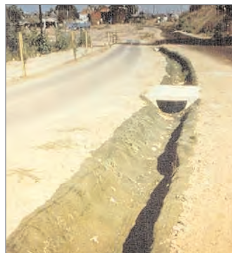
Figure 18.9 Left: diversion drain alongside sloping pipeline easement (courtesy Alfred McAlpine)
