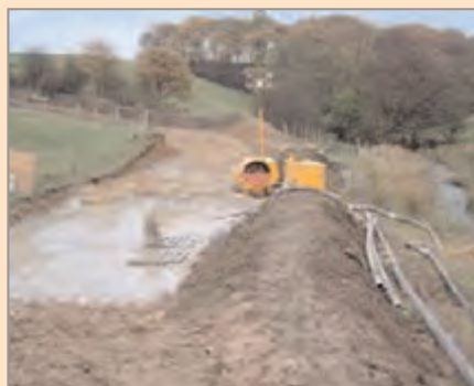
Figure 20.9 Grout emerging from borehole into lagoon
