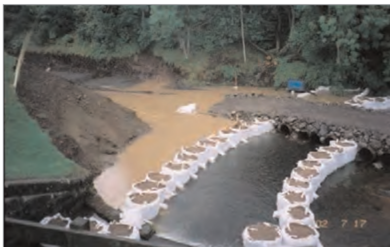
Figure 20.12 Silt trap comprising bags of sand used during watercourse diversion (courtesy Balfour Beatty)
