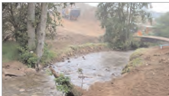
Figure 20.16 Timber boards and coir matting installed as river bank stabilisation (courtesy Transco)
