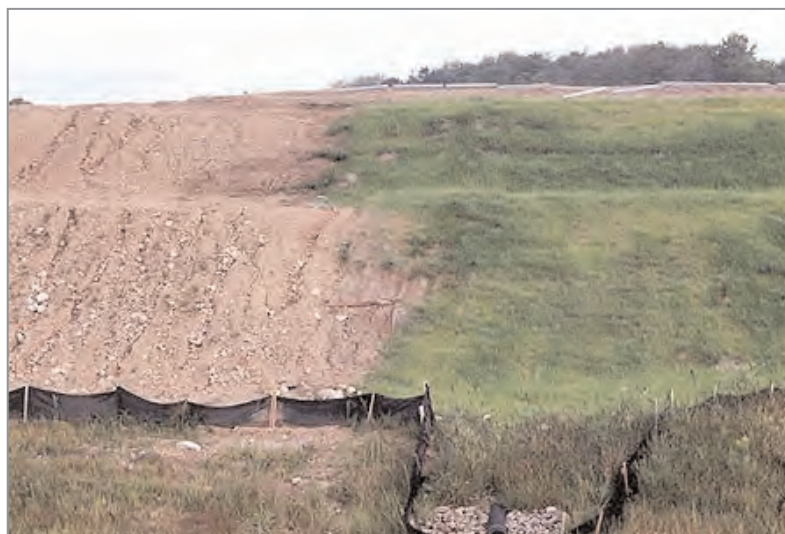
Figure 18.3 Before and after seeding: erosion gulleys on non-vegetated slope (courtesy IECA)
