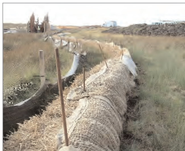
Figure 18.18 Silt fence and straw bale arrangement to control silty runoff; note buffer zone between fence and earthworks (courtesy Mowlem)
