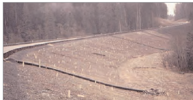
Figure 18.12 Slope drain (Oregon DEQ, 2004)
