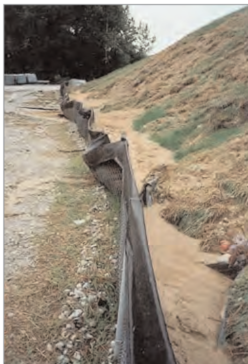
Figure 18.15 Fabric silt fence at toe of stockpile (courtesy IECA)
