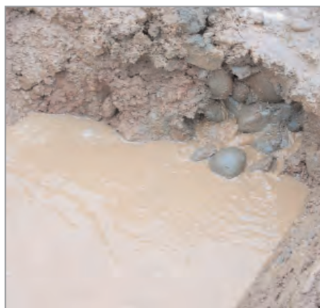
Figure 18.21 Above: land drain uncovered during construction work (courtesy Transco)
