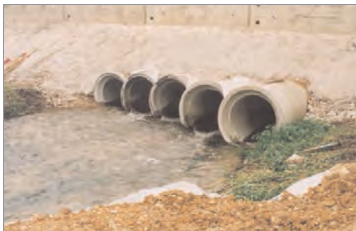
Figure 20.5 Haul route culverts sized for maximum flood flow (courtesy Costain)
