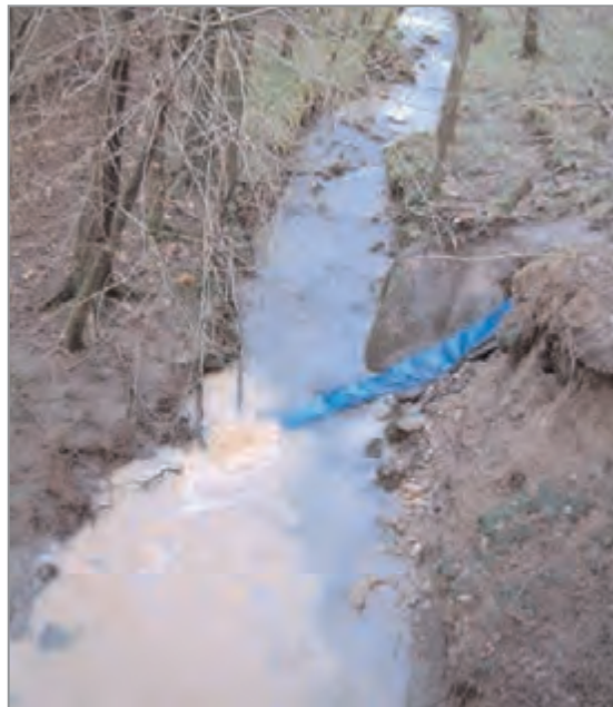
Figure 21.1 Discharging water from pumping activities has caused silt pollution in the stream
