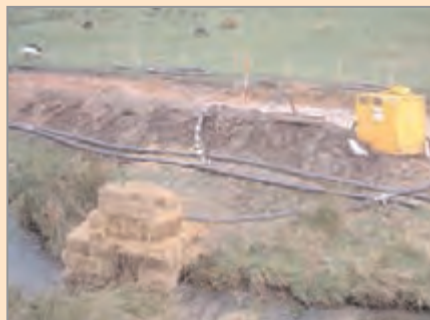
Figure 20.10 Clean discharge from lagoon entering stream through straw bales
