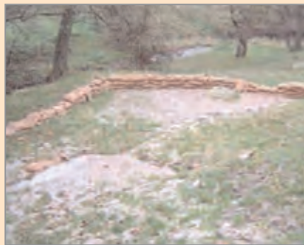
Figure 20.7 First grout breakout controlled with sand bags
