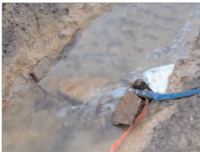
Figure 20.14 Large stones used for bed protection at a pipe outfall
