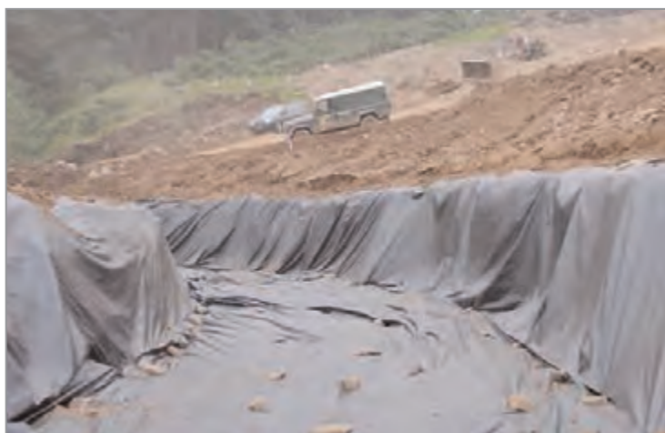
Figure 20.13 River diversion to allow open-cut crossing. Lined with geotextile to avoid silt generation (courtesy Entrepouse)
