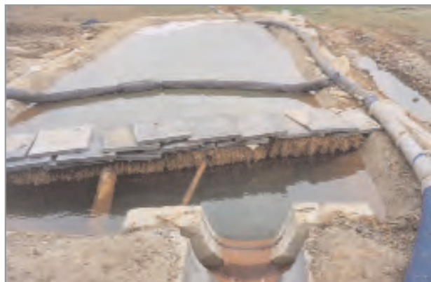
Figure 19.6 Settlement pond with straw bale filter and oil boom (courtesy Hyder). Note that fluctuation of the water level has lifted the ends of the boom above the water surface, which might allow oil to flow underneath
