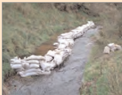
Figure 20.8 Second breakout controlled with sand bags in stream
