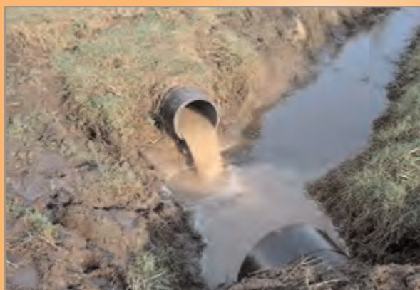
Figure 19.1 Silty water discharging through land drain into ditch (courtesy Transco)
