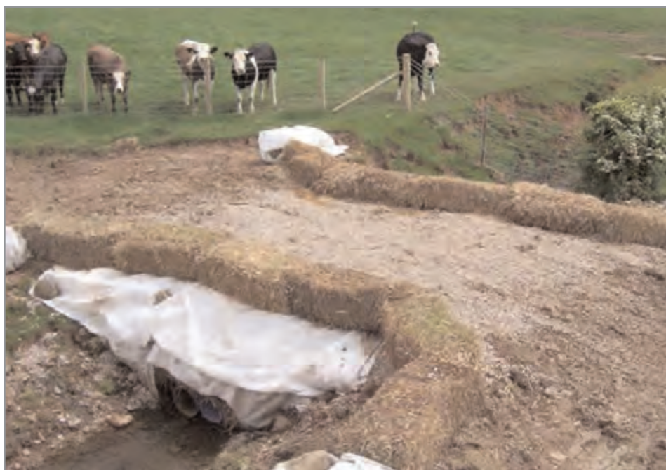
Figure 20.4 Culverted haul route crossing (note straw bales and geotextile to filter silty runoff) (courtesy Morgan Est)
