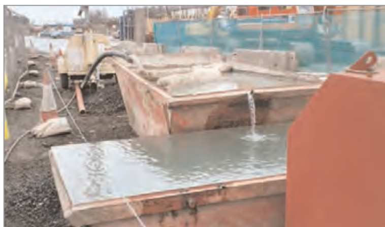
Figure 19.5 Skips used as settlement tanks (courtesy Hyder)
