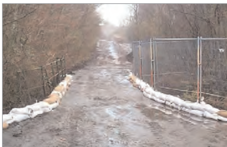
Figure 20.6 Sand bags along existing bridge protecting river below from haul road runoff (courtesy Morrison Construction)
