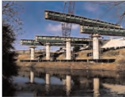
Figure 20.18 Beams for the M1A1 bridge being erected over the River Aire (courtesy Balfour Beatty)
