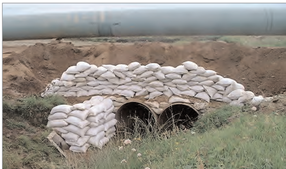
Figure 20.11 Flume pipes carrying water flow during open-cut crossing of stream for pipeline installation (courtesy Transco)
