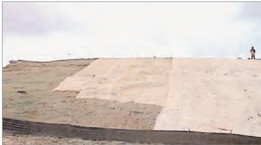
Figure 18.5 Coconut matting and silt fence (Oregon DEQ, 2004)
