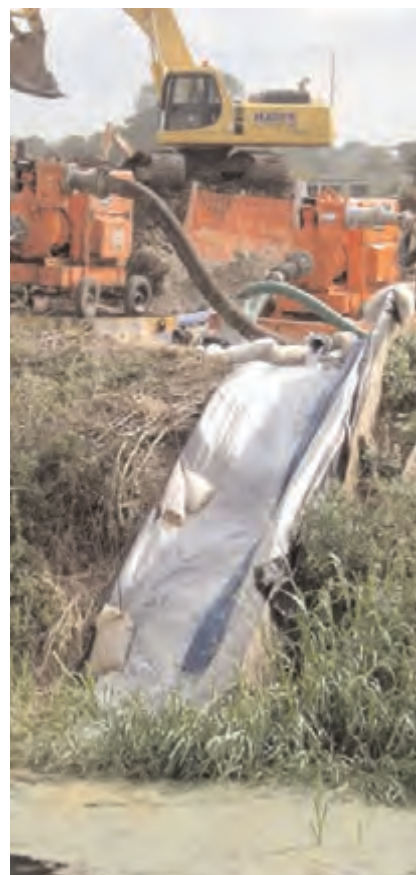
Figure 19.8 Right: bank protection for discharge outfall (courtesy Transco)
