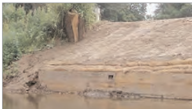
Figure 20.16 Timber boards and coir matting installed as river bank stabilisation (courtesy Transco)
