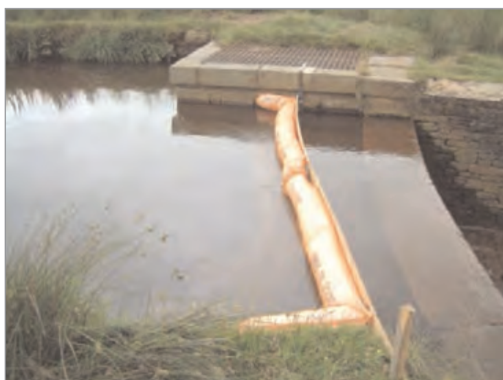
Figure 20.3 Correct installation of oil boom
