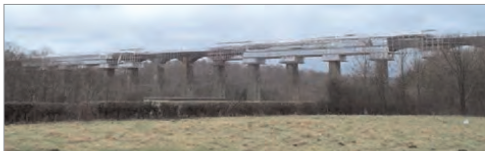
Figure 20.17 Sheetting of Pontcysyllte Aqueduct over River Dee SSSI (courtesy British Waterways)
