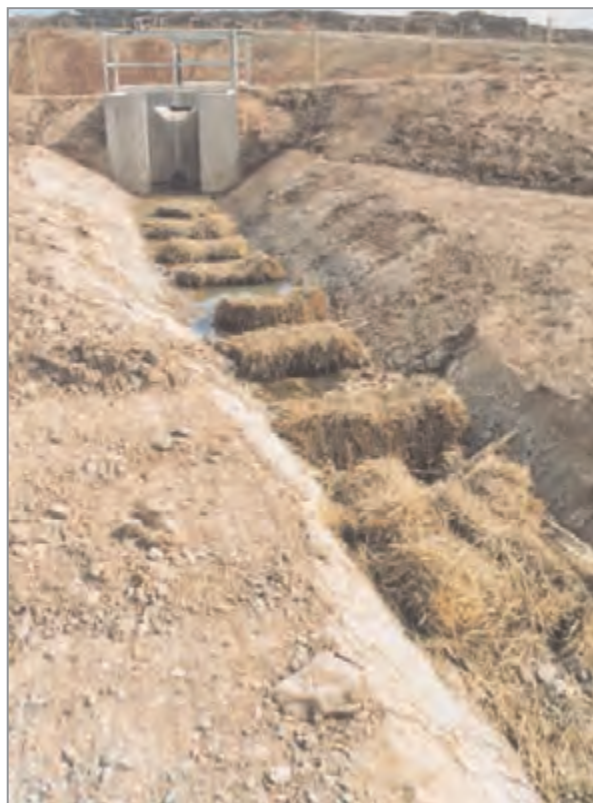
Figure 20.1 Straw bales filtering silt in a newly constructed stream (courtesy Hyder)
