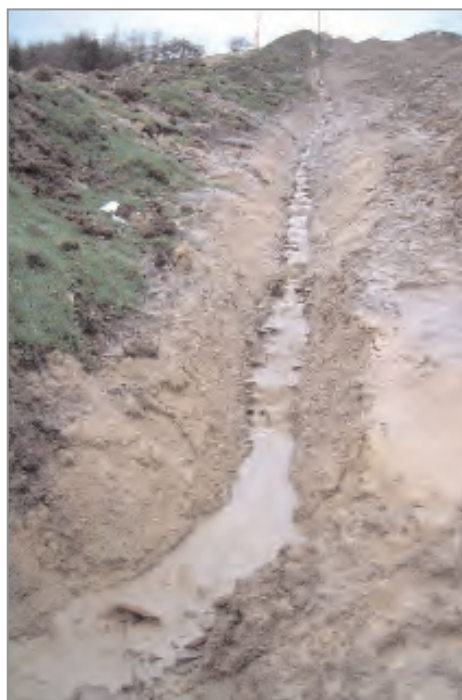
Figure 18.9 Left: diversion drain alongside sloping pipeline easement (courtesy Alfred McAlpine)
