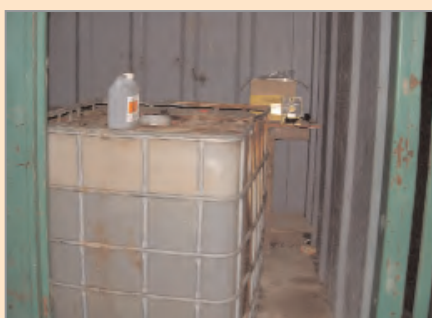
Flocculant dosing pump and IBC inside steel cabin
