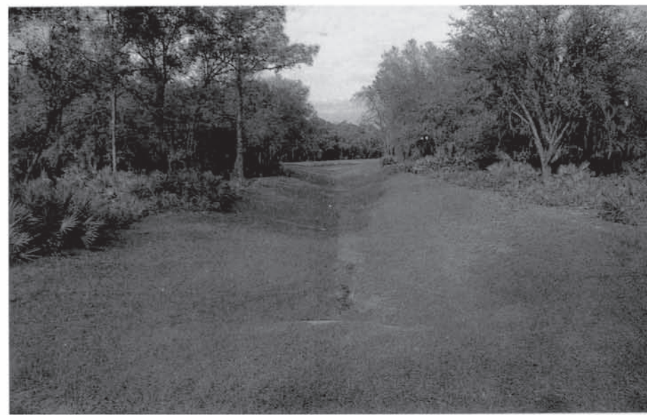
Swale Discharge From Wetland
