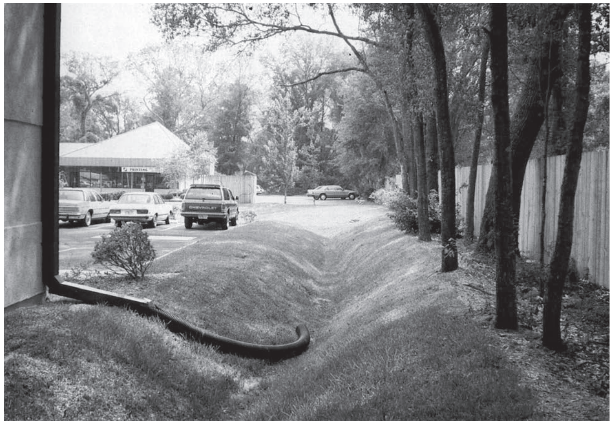
Infiltration Practice: Directing runoff to grassed areas.
