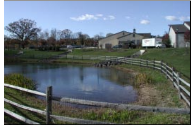
Wet detention basins planted with appropriate plant material can improve the look and function of the basin.
