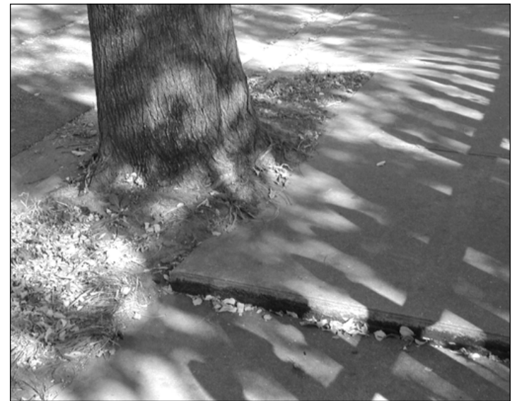
A buckled sidewalk is a lawsuit waiting to happen. This sidewalk should have been placed farther from the tree. To reduce liability now without removing the tree, the sidewalk could be moved slightly.
