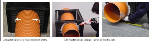
Apply sealant around the pipe to cover all possible leaks
