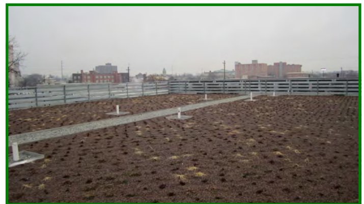
Extensive green roof with non-vegetated access path and buffers around vents (Photo: Erin Wagoner, URS)
