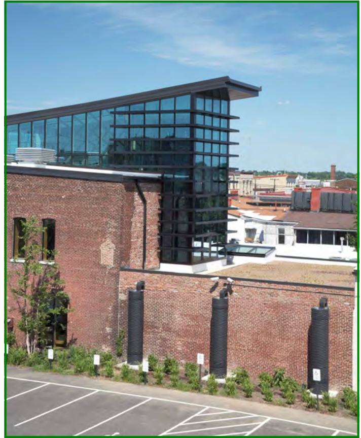
Three cisterns capture and store excess runoff from rooftop surfaces at the Green Building and are drained between rain events to water the bioswale and rain garden. (Photo: Ted Wathen)
