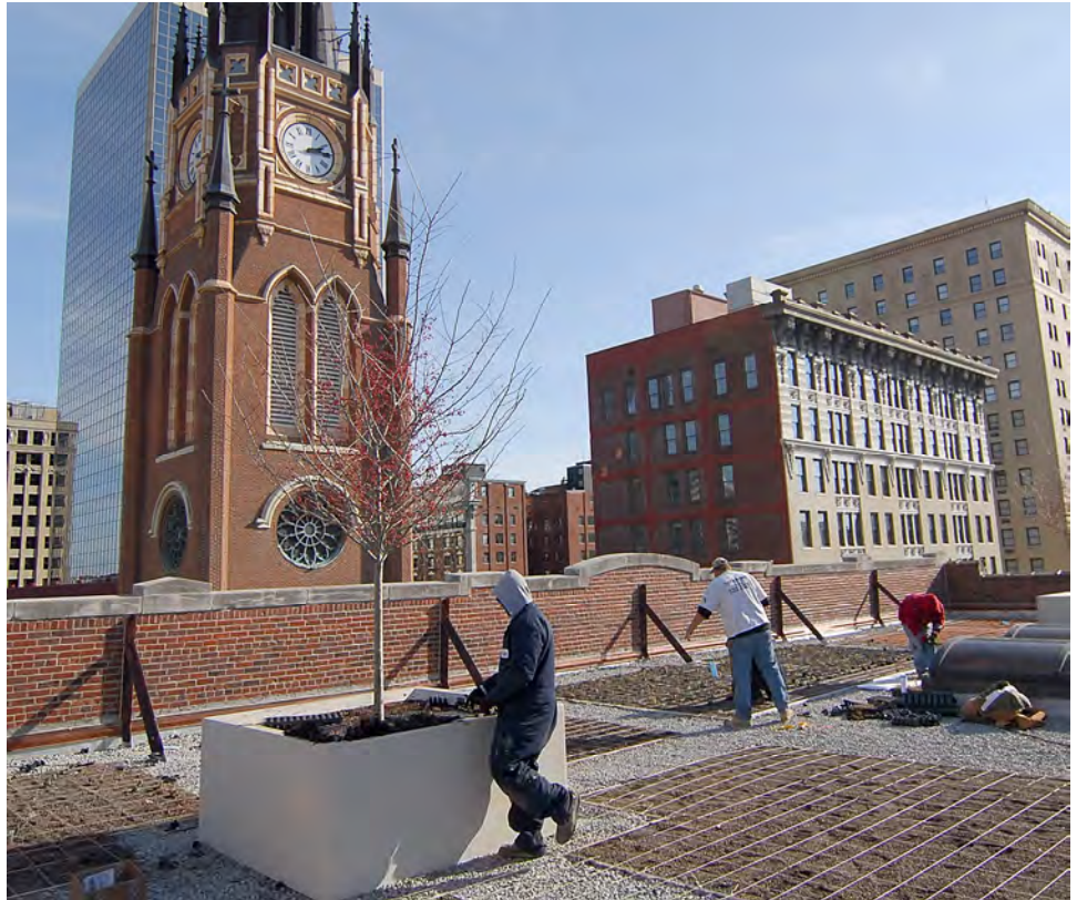
Intensive (deep) and extensive (shallow) green roof beds (Photo: Louisville & Jefferson County MSD)
