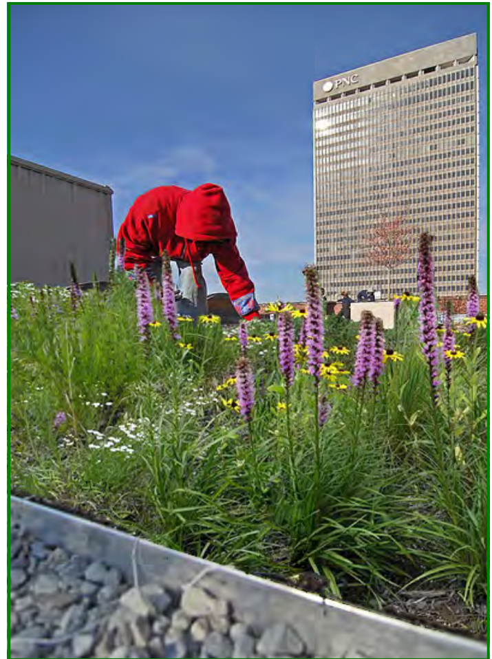
Remove sediment, trash, weeds and debris (Photo: Louisville & Jefferson County MSD; Concept Rendering: Shea Powell, Dropseed Nursery)
