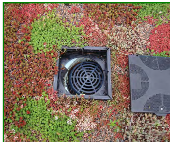
Established sedum plants on extensive green roof (Photo: Chad McCormick, URS)
