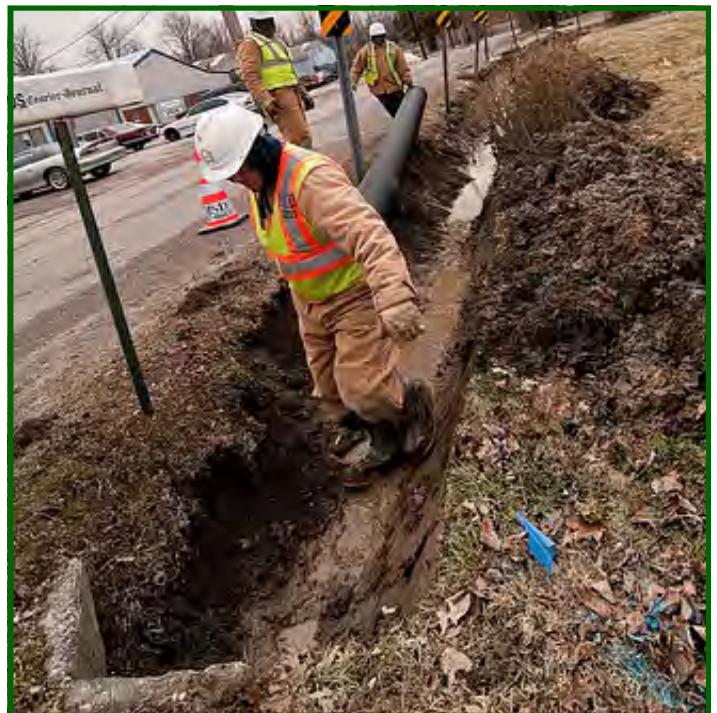
Installation of a new drainage system along Reynolds Avenue (Photo: Louisville & Jefferson County MSD)
