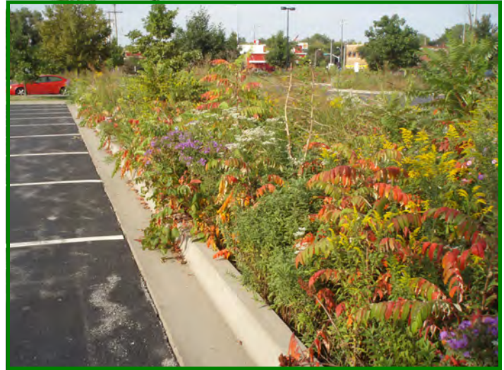
Bioswale with naturalized, established native plantings (Photo: David Dods, URS)
