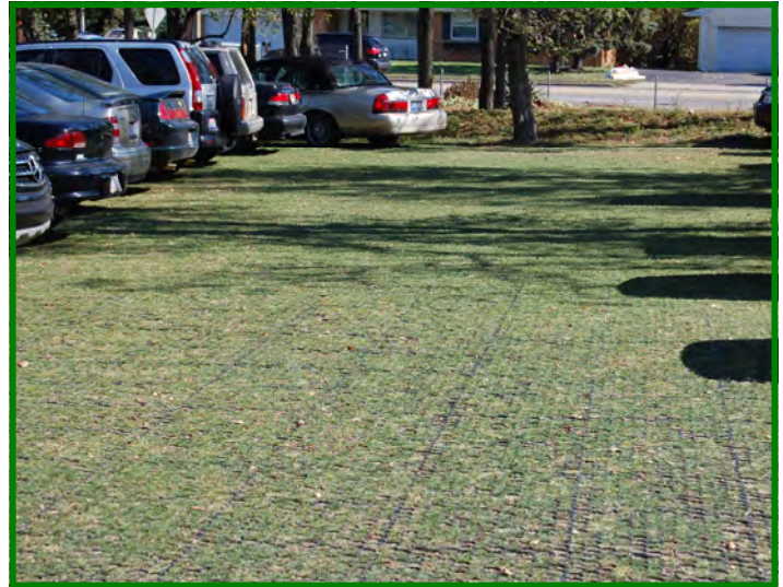
Grass pavers used in a church parking lot (Photo: Site Supply, Inc)
