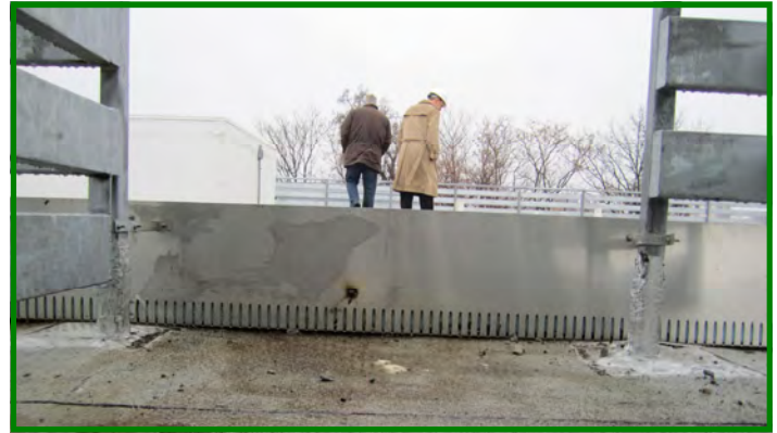
Extensive green roof showing drainage slots and non-vegetated buffer along roof perimeter (Photo: Erin Wagoner, URS)
