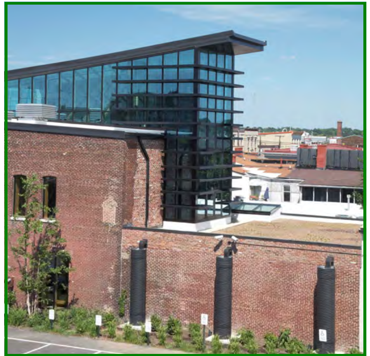
Stormwater treatment train flows from green roof to cisterns to a bioswale (Photo: Ted Wathen The Green Building)
