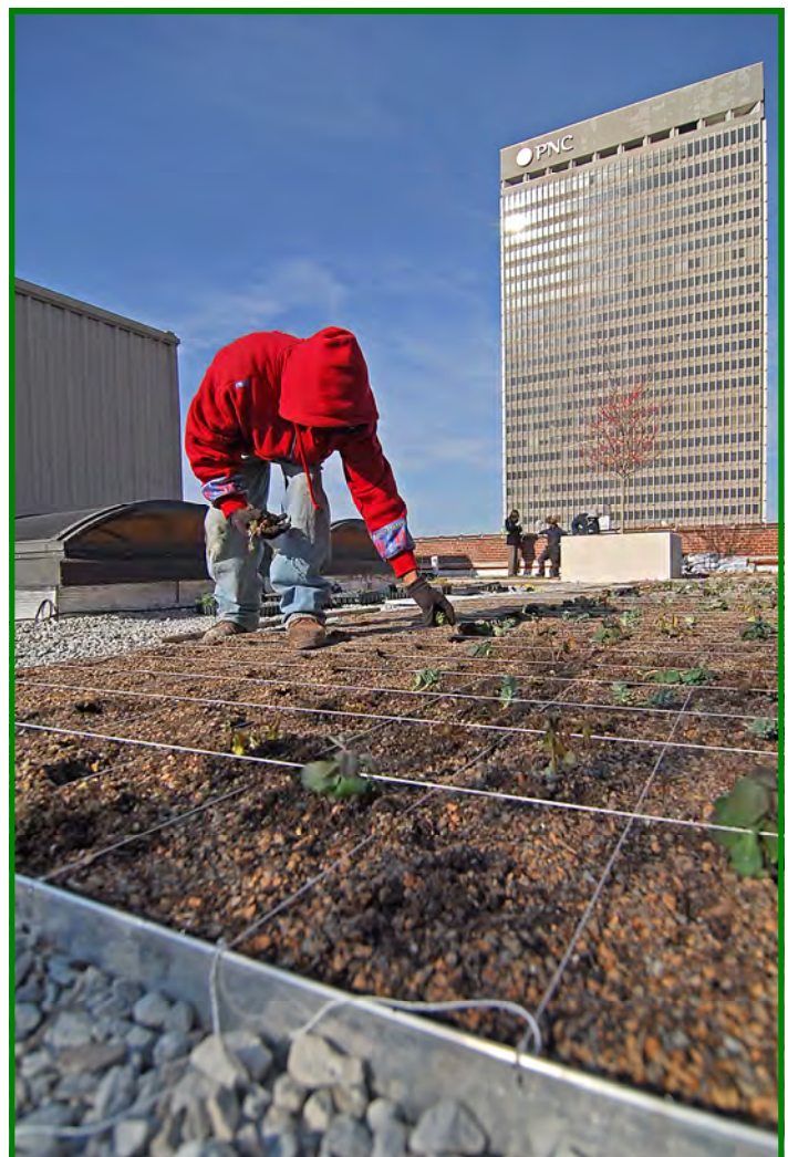
Installation of plants on an extensive green roof (Photo: Louisville & Jefferson County MSD)
