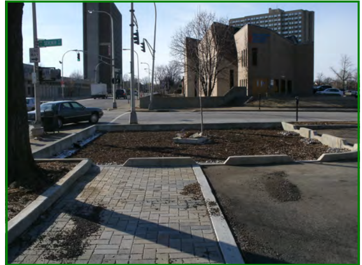
Permeable pavers should be inspected for trash, debris and dirt (Photo: Bethany Shain, URS)
