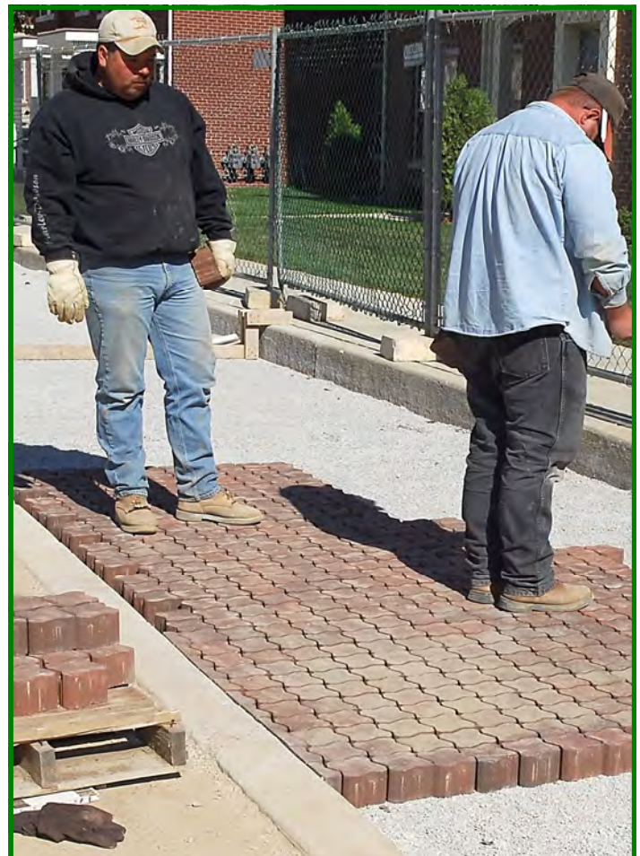
Installation of permeable interlocking concrete pavers (Photo: Louisville & Jefferson County MSD)
