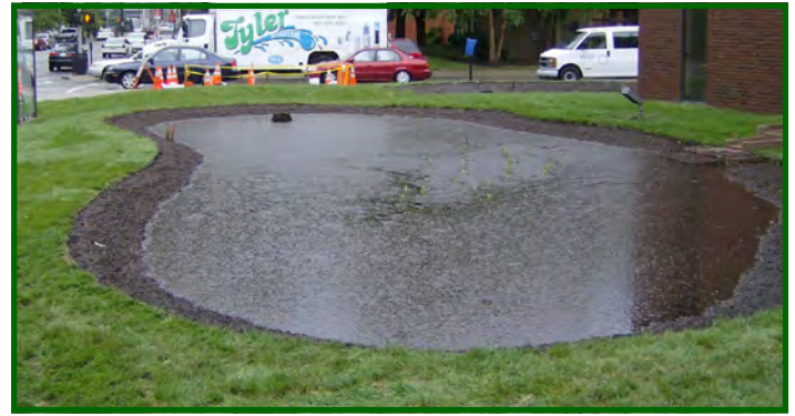
MSD rain garden at 700 West Liberty Street immediately after installation (Photo: Louisville and Jefferson County MSD)
