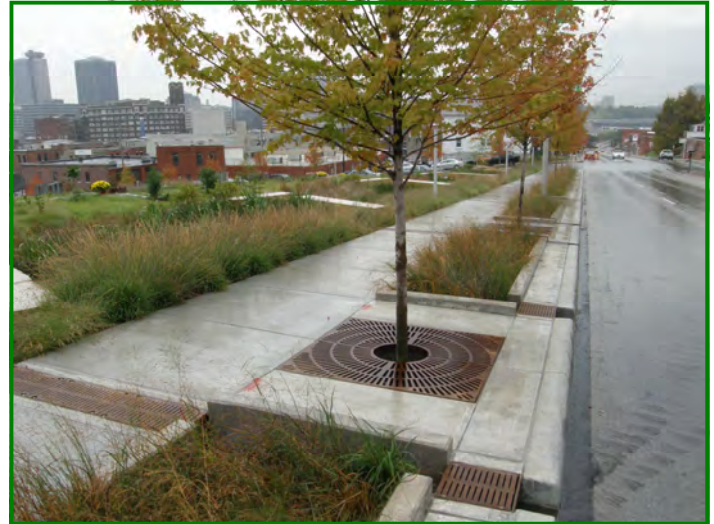
Series of tree and planter boxes accept stormwater runoff from a roadway and should drain within 24 hours after the rain event (Photo: David Dods, URS)
