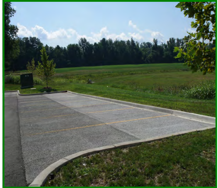
Pervious Concrete Parking Spaces at Dixie Highway Kroger in Louisville KY. (Photo: Erin Wagoner, URS)
