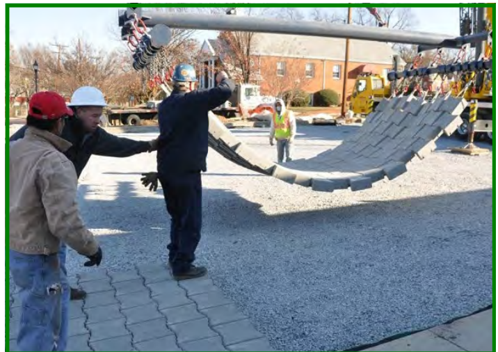
Installation of articulated concrete block mats (Photo: Site Supply, Inc)
