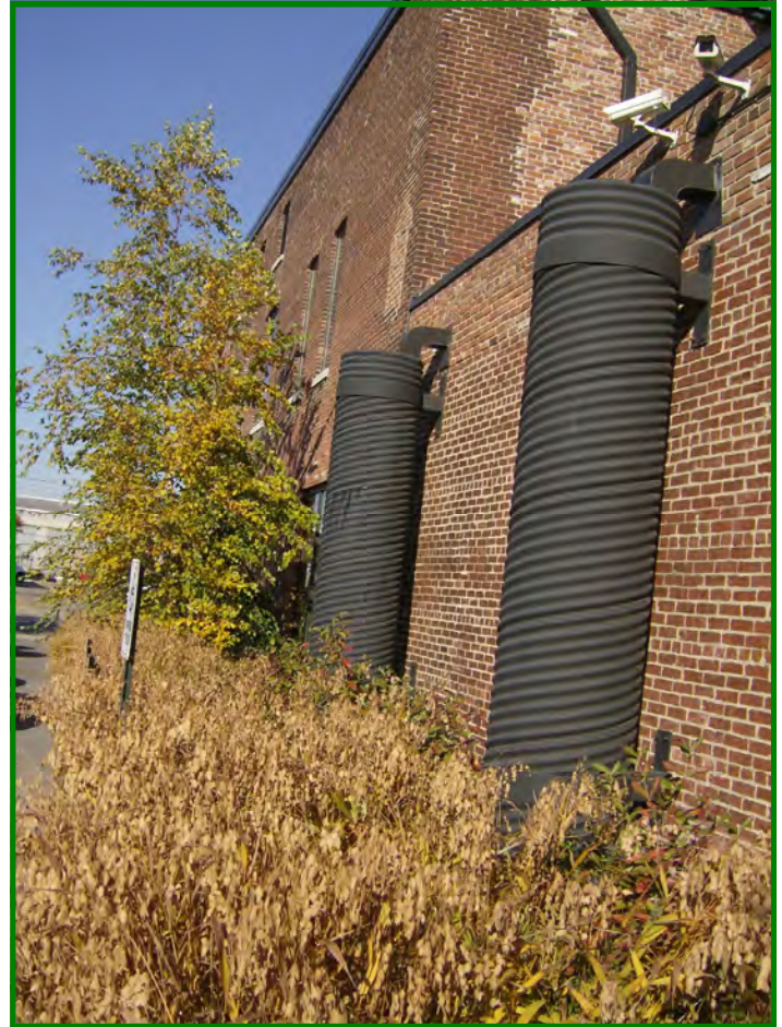
Rainwater harvesting cisterns at the Green Building (Photo: Erin Wagoner, URS)
