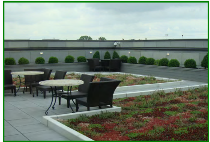
Extensive green roof beds (foreground) are paired with intensive green roof beds (background), planted with evergreen shrubs (Photo: Chad McCormick, MSD)
