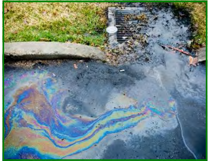
Catch basins should be kept free of sediment, trash and debris. (Photo: Dauphin County Conservation District, Pennsylvania)
