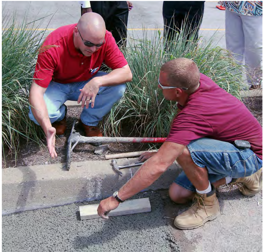
Installation of Pervious Concrete (Photo: Louisville & Jefferson County MSD)
