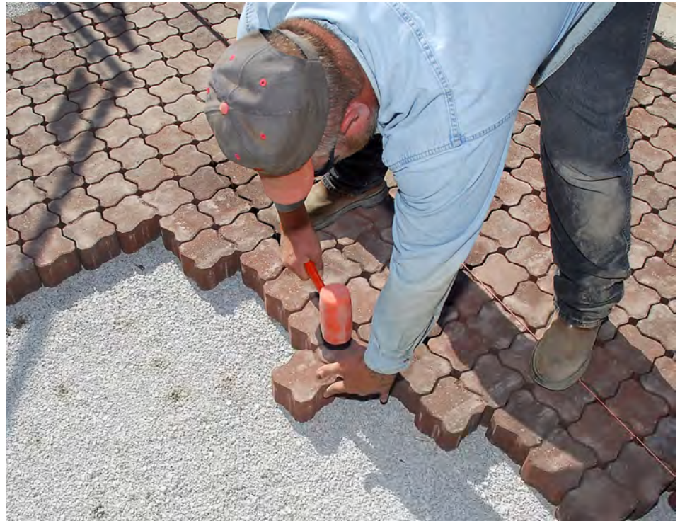
Installation of permeable interlocking concrete pavers (Photo: Louisville & Jefferson County MSD)
