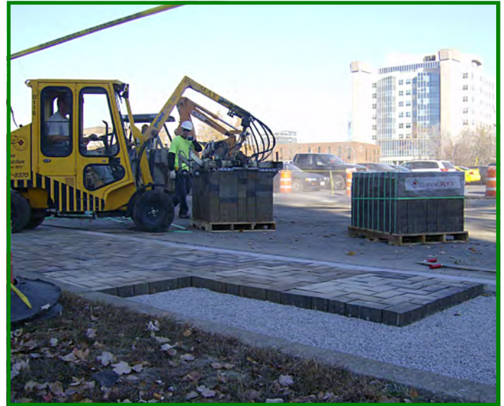
Mechanical installation of permeable interlocking concrete pavers (Photo: Erin Wagoner, URS)
