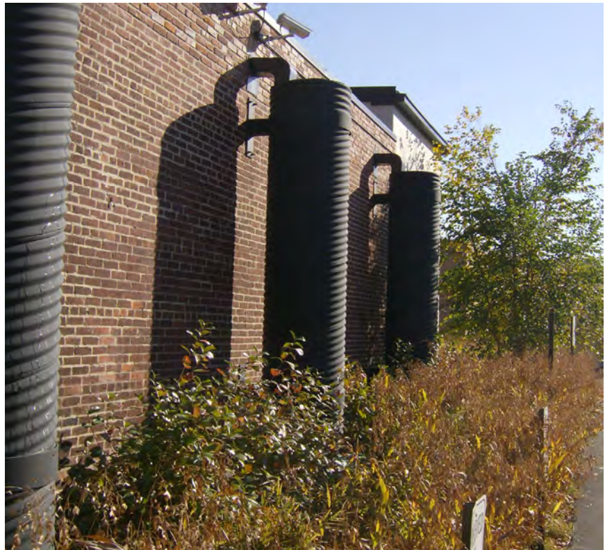
Cisterns drain to a bioswale at the Green Building in Louisville (Photo: Erin Wagoner, URS)
