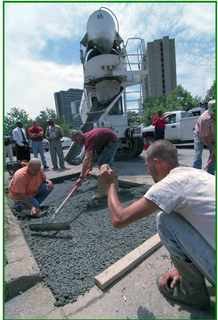
Installation of pervious concrete (Photo: Louisville & Jefferson County MSD)
