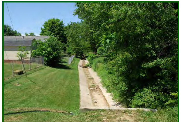
Concrete lined drainage way in Louisville Metro (Photo: Louisville & Jefferson County MSD)
