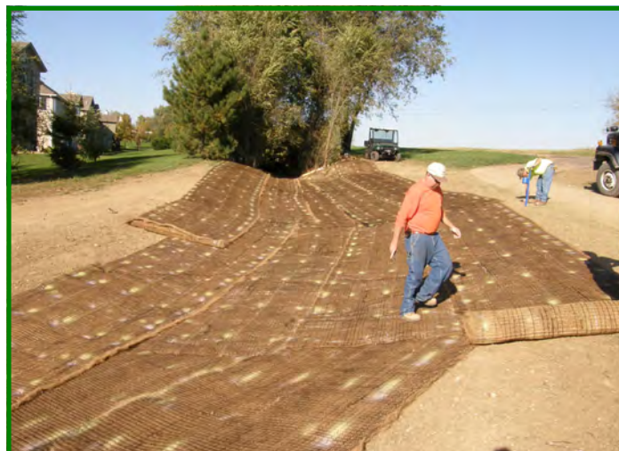
Vegetated swale installation using turf reinforcement mats (Photo: David Dods, URS)
