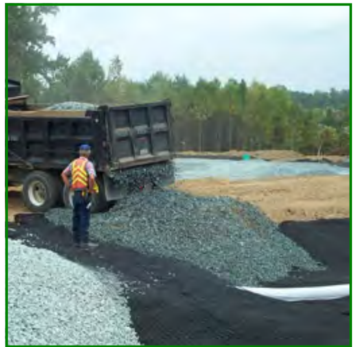
Stone Reservoir with Drainage Pipes (Photo: CH2M Hill)
