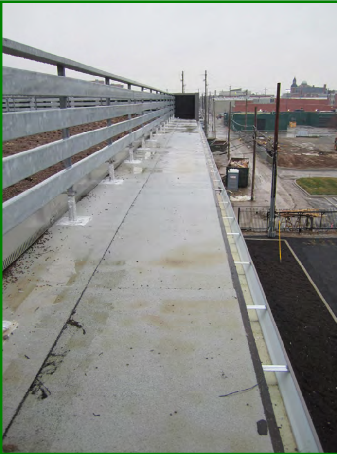
Excess drainage from extensive green roof flows from drainage layer slots over non-vegetated buffer to roof downspouts, which discharge into a rain garden (Photo: Erin Wagoner, URS)
