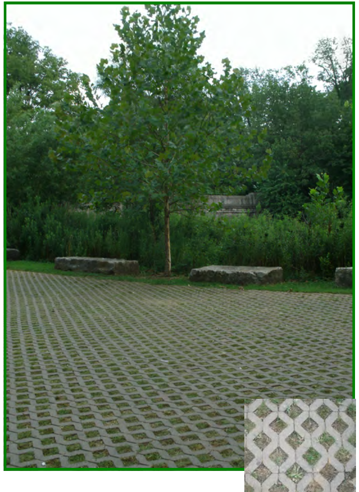
These permeable pavers in a parking lot at Cherokee Park are concrete grid permeable pavers, consisting of a grid filled with topsoil and planted with grass. Concrete grid permeable pavers should be used for light traffic use, such as this overflow parking lot. (Photos: Erin Wagoner, URS)
