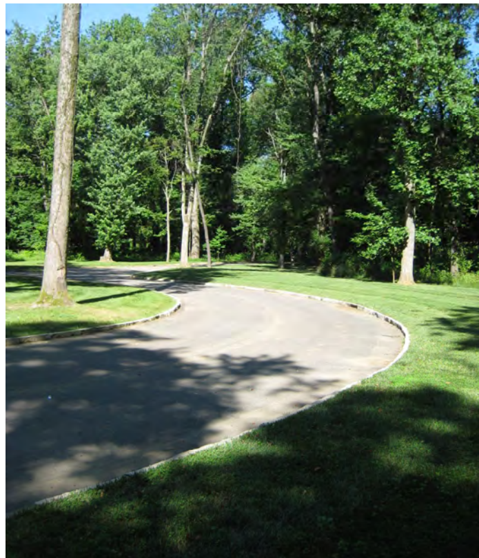
Figure 18.3-F. This residential street in a development using conservation and open space design uses narrower streets than traditional practices. (Photo Sabak, Wilson and Lingo Inc.)
