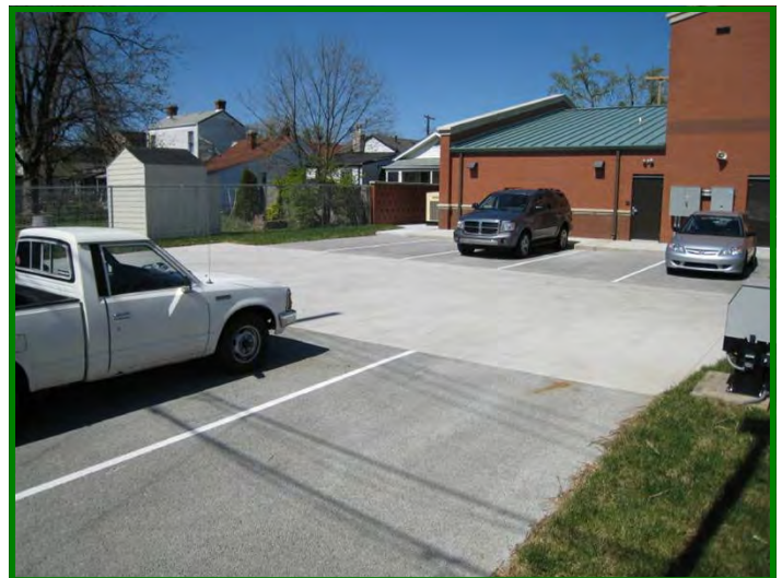
Pervious concrete at Louisville Fire Station (Photo: Kentucky Concrete Pavement Association)
