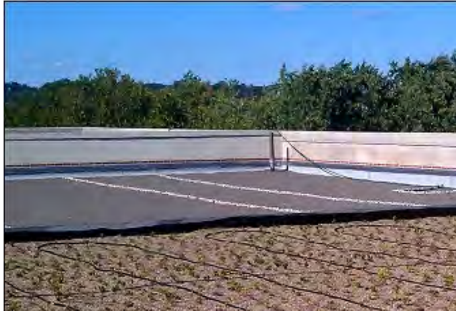
Blue roof adjacent to green roof (Photo: New York City Blue Roof and Green Roof Comparison Study)
