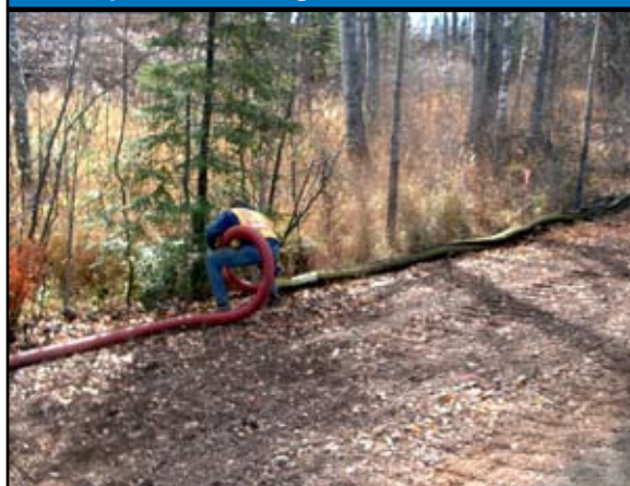
Figure 14.12 Perimeter Control Using Compost Filter Logs
