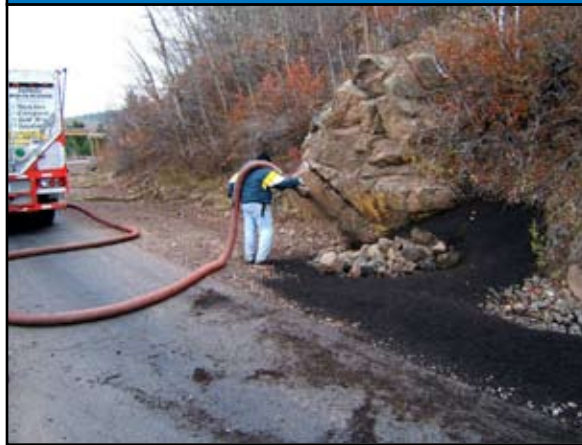
Figure 14.14 Compost Soil Amendment for Rapid Vegetation and Stabilization
