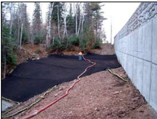
Figure 14.15 Rapid Stabilization and Revegetation Using Compost and Vegetative Mat (a) Installation and (b) After Stabilization (Note that areas utilizing compost vegetated more quickly and completely than areas using the vegetative mat.)
