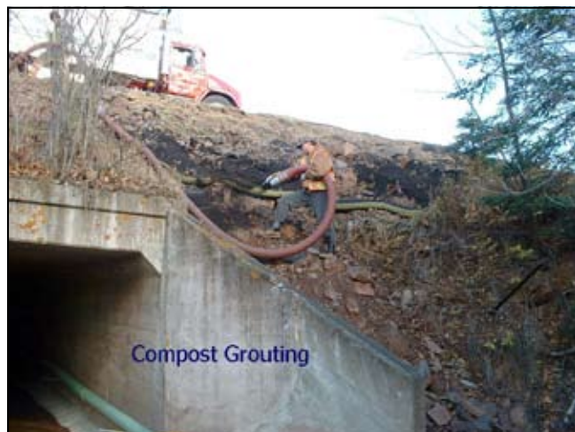
Compost grouting on Highway 61.
