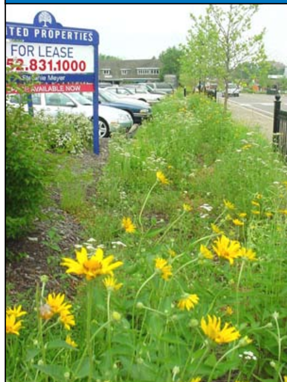
Figure 12.FIL.2 Vegetated Swale (Wayzata, MN)
