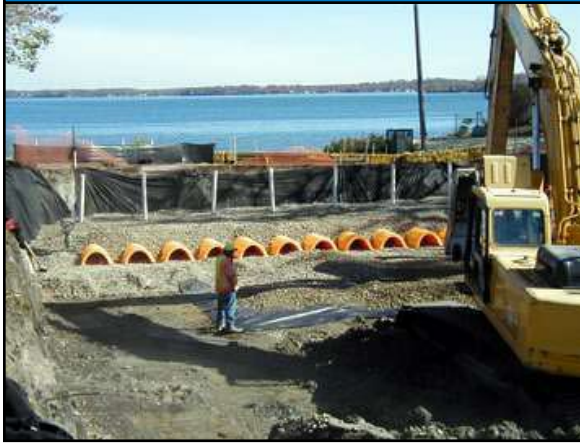
Figure 14.24 Filtration System Installation
