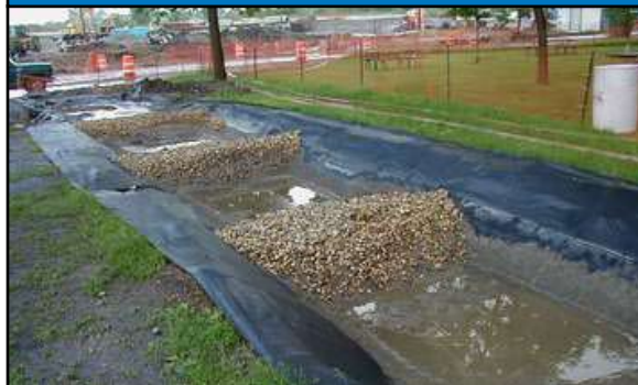
Figure 14.23 Temporary Sedimentation Basin
