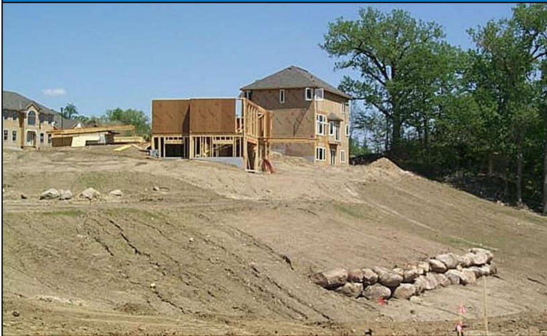
Figure 2.3 Uncontrolled Construction Erosion
