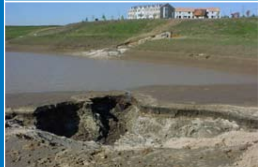
Figure 13.2 Collapsed Karst Feature
