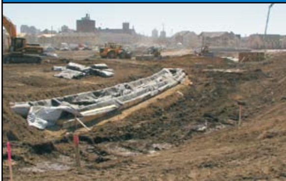
Figure 14.7 Installation of Trench Forebay
