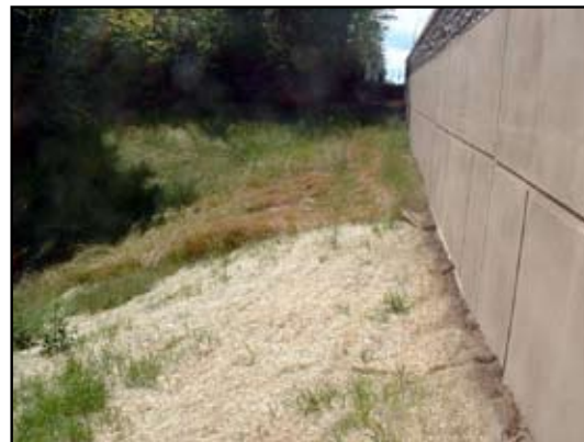
Figure 14.15 Rapid Stabilization and Revegetation Using Compost and Vegetative Mat (a) Installation and (b) After Stabilization (Note that areas utilizing compost vegetated more quickly and completely than areas using the vegetative mat.)
