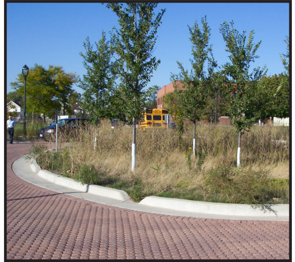
Figure 1.5 Rain garden in roundabout designed to capture/infiltrate stormwater, Milwaukee, WI. Source: Bob Newport, EPA Region 5
