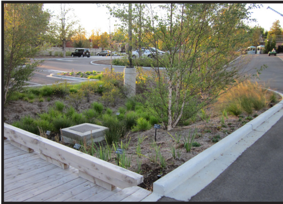
Parking lot with rain garden and overflow, plus permeable pavement and curb cutouts above. Source: Metropolitan St. Louis Sewer District
