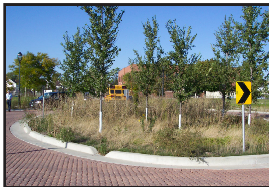
Figure 2.13 Rain garden in roundabout designed to capture/ infiltrate stormwater, Milwaukee, WI. Source: Bob Newport, EPA Region 5
