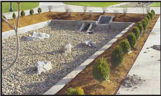
Sand Filter (Open Basin Design)- North Carolina. Source: North Carolina Stormwater BMP Manual .
