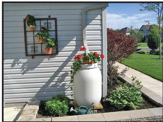
Figure 2.14: Residential rain barrel. Source: ABCs of BMPs
