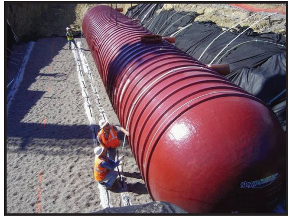
Installation of the water harvesting cisterns.
