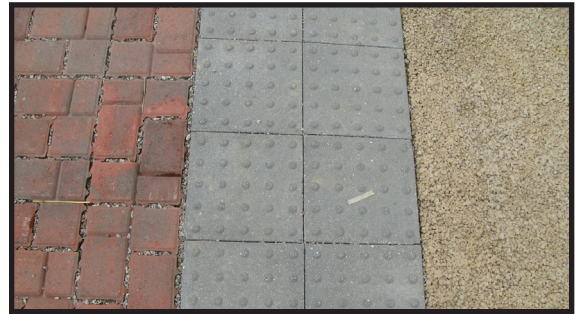
Figure 6.27 Pervious pavement types. Source: Williams Creek Consulting.
