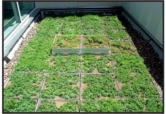
Figure 6.5 Extensive Green Roof- University of Missouri, Life Science Center- Columbia, MO. Source: www.greenroofs.org
