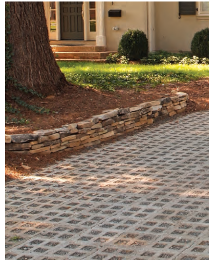
Eco-Grid pavers, filled with recycled gravel
