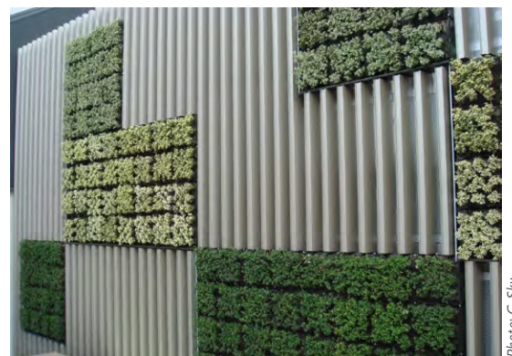
Recycled Steel Green Screen
