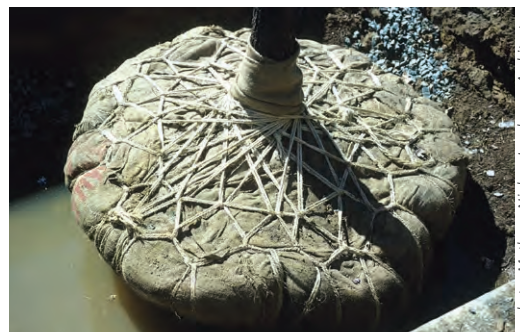
New tree installed in tree pit. Structural soil backfill facilitates air and water movement
