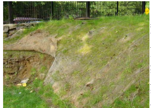
Erosion control fabric and vegetated slope protection at Riverdale Country School
