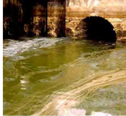
Combined sanitary/stormwater sewer outfall
