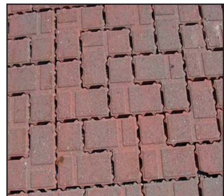
Figure 2.11.7 Pervious Interlocking Concrete Pavement
