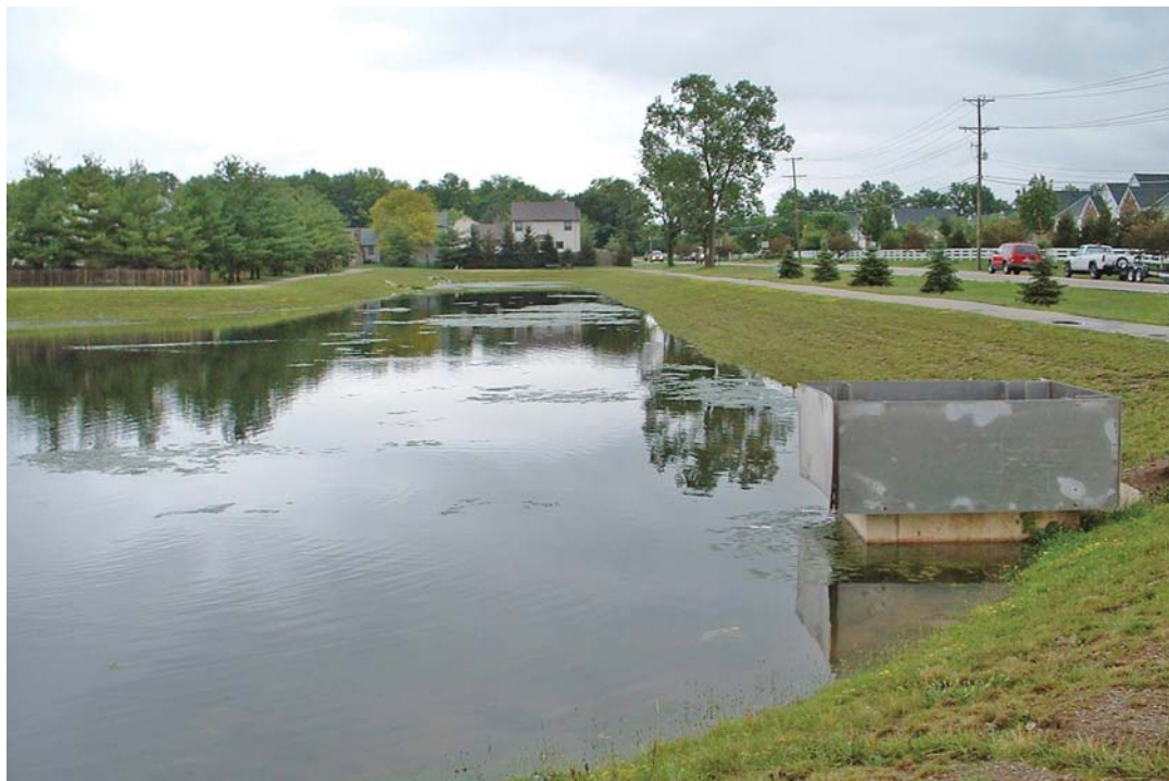
Wet extended detention pond
