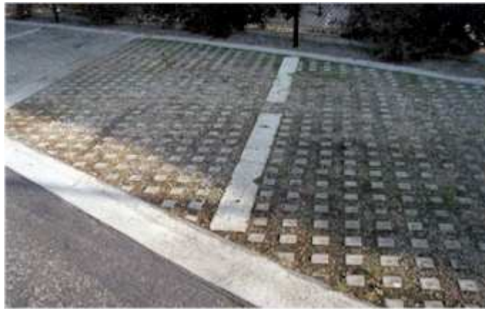
Figure 5.10-2 Overflow parking using permeable pavers
