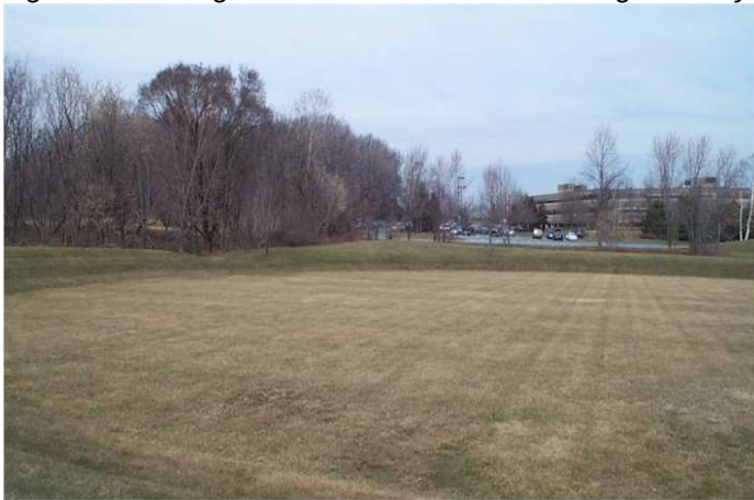
Figure 9-11. Vegetated infiltration basin in Lehigh County.
