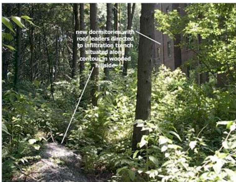
Figure 9-27. Level spreader pipe/infiltration trench in woods.
