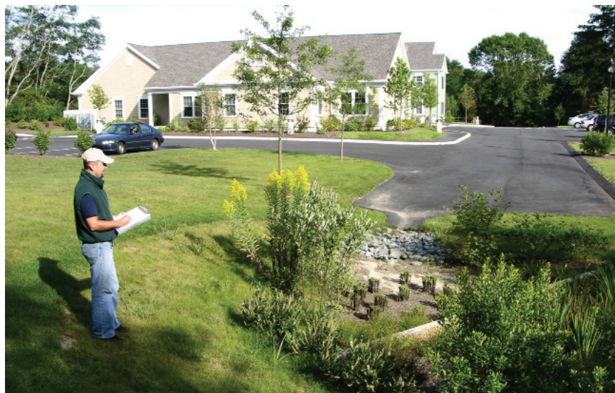
Figure 9-6 Inspection of Bioretention Facility.
