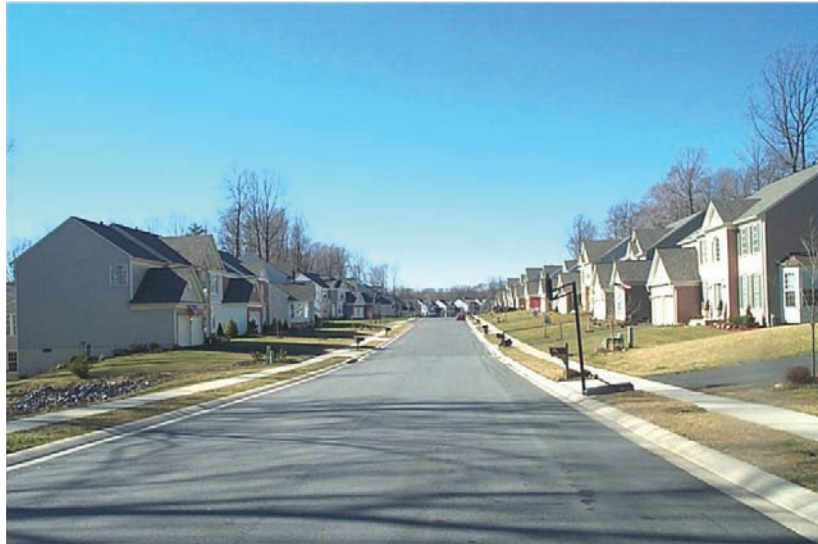
Figure 5-1 Excessive Roadway Design.
