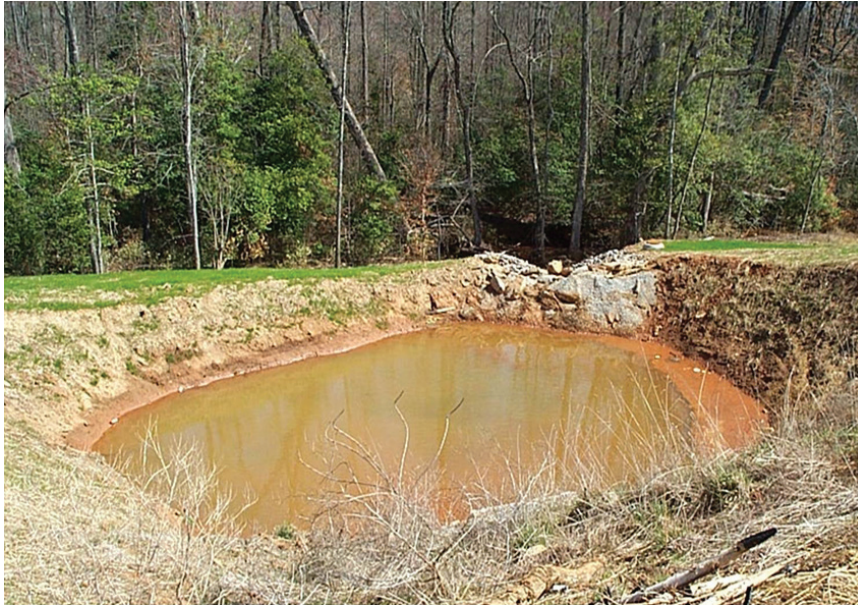
Figure 9-4 Properly Installed Erosion and Sediment Control Practice.
