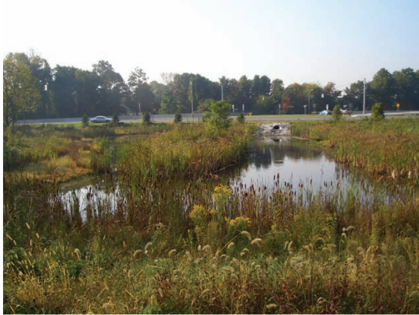
Figure 9-9 Stormwater Facility Requiring Regular Inspection.
