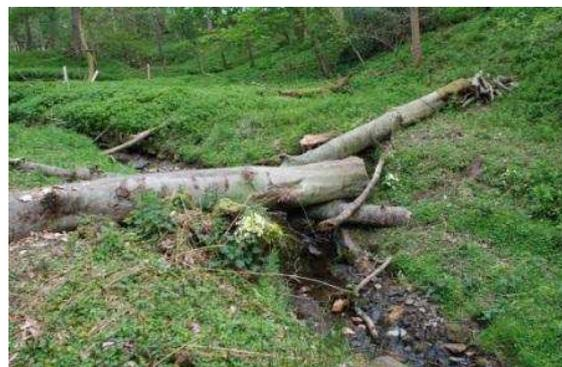
*Figure 22 – Timbers placed in cross formation*
