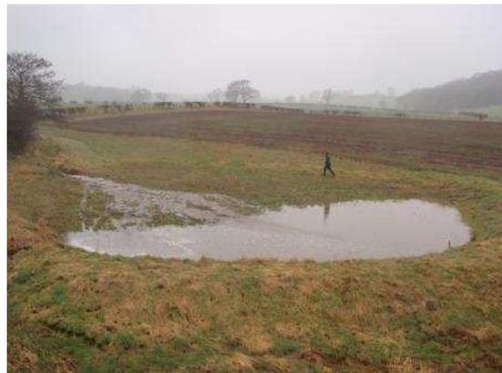
*Figure 8 – Offline pond starting to fill during heavy rain*
