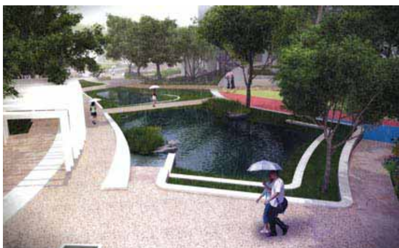
Figure 6.1.5 Bioretention basin serving as a multi-purpose lawn during dry weather. During a rain event, it acts as a temporary detention feature for stormwater runoff.
