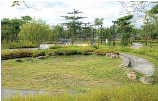
Figure 3.13 Dry pond at Greenwood Sanctuary - During rain events, stormwater runoff flows from the surrounding ground to the dry pond and filters to underground percolation tanks encased in a permeable membrane layer. During dry weather, the lawn area in the dry pond can also be used for recreational activities.
