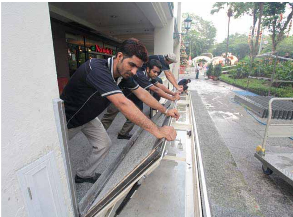
Figure 5.7 Regular tests and inspections of flood barrier systems are necessary to ensure that the system can be reliably activated during flood events.
