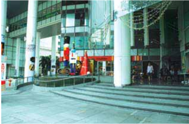
Figure 4.3 Steps and ramps are some of the options to achieve the minimum platform levels for developments with entrances to underground facilities.
