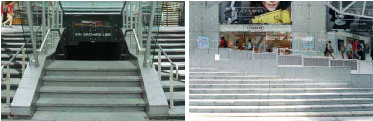
Figure 4.4 Additional crest protection levels are required for developments with underground linkages to MRT stations (e.g. Ion Orchard Link) and for all openings to basement facilities, including ventilation ducts (e.g. Wisma Atria)
