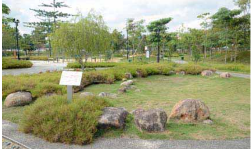
Figure 5.3 Using a combination of gradual slopes and clear signage, this dry pond allows users to move out of the area safely and easily during a rain event.
