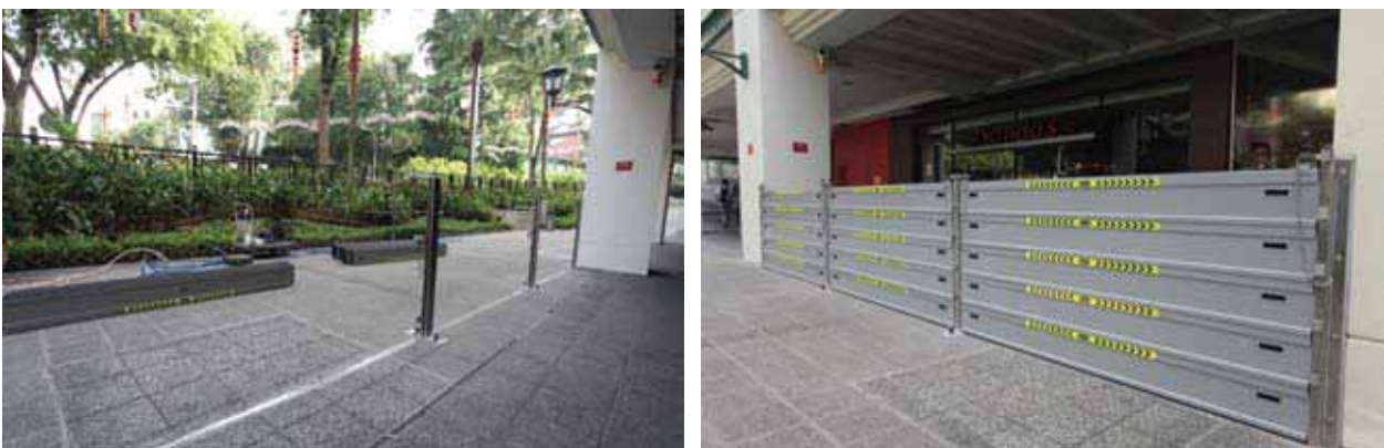
Figure 6.2.4 A multi-slot barrier at the front of Tanglin Mall before (left) and after (right) installation. These barriers have to be installed manually.
