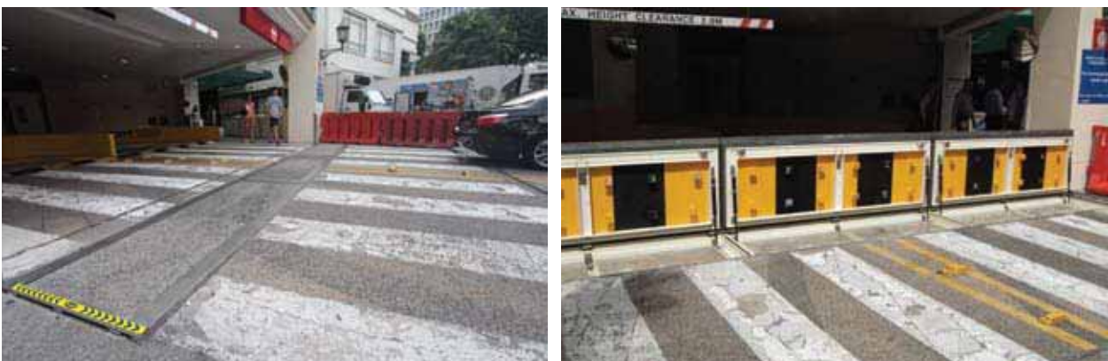
Figure 6.2.3 A flip-up barrier at the entrance to the basement carpark in closed (left) and open (right) positions.
