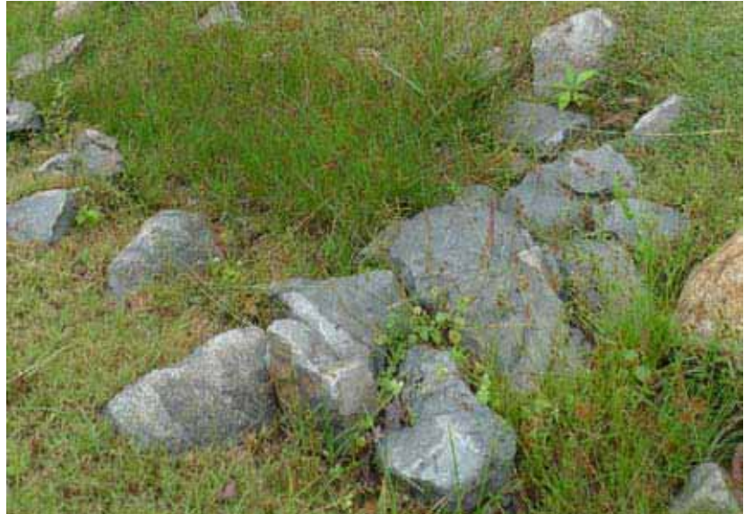
Figure 5.6 Sedimentation and excessive vegetation have grown inside the swale, obstructing flow and reducing conveyance capacity during rain events. This could also potentially be a breeding ground for mosquitoes when stagnant water is trapped in the swale. Regular maintenance of the swale is required to ensure its functionality.
