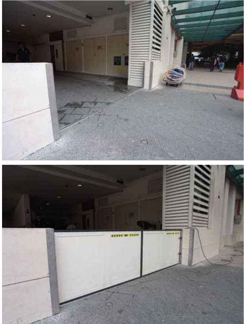
Figure 6.2.5 Swing-type flood barrier in open (top) and closed (bottom) positions at access to loading/unloading areas.
