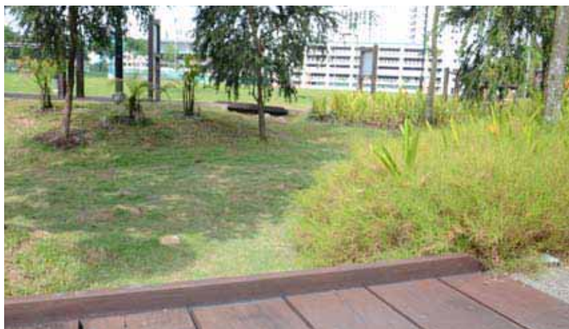
Figure 5.5 Erosion in grass swales can be minimised by planting more resilient or water-tolerant species in areas that experience higher flow velocities or are frequently submerged (e.g. depression areas).
