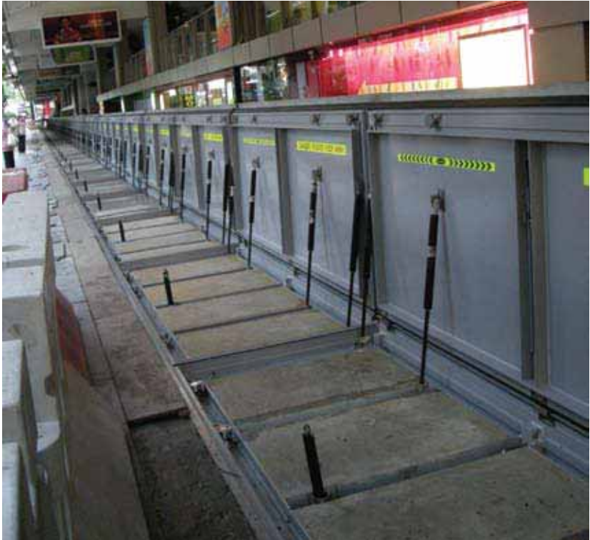
Figure 4.17 Automatic flood barrier system at Lucky Plaza.
