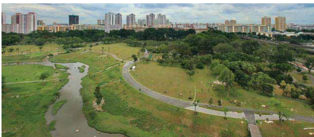
Figure 1.8 Acting both as a pathway and source solution along Kallang River, Bishan-Ang Mo Kio Park is an integrated multi-functional space that provides active recreational spaces for park users during dry conditions, but morphs into a floodplain during rain events, providing additional drainage capacity for the waterway.
