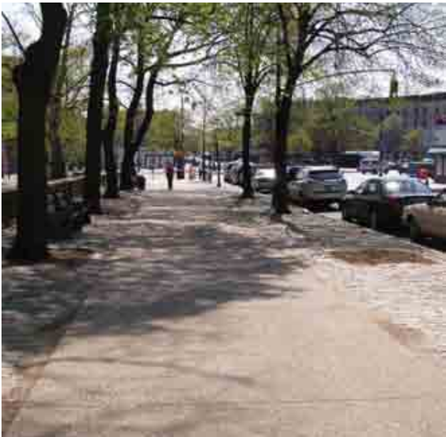
Sand-colored concrete sidewalk with exposed aggregate: Prospect Park West, Brooklyn
