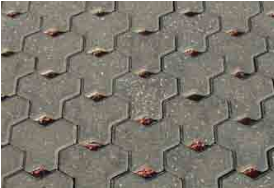
Voids between pavers allow rainwater to trickle through: Bicentennial Park, Sydney, Australia (Credit: Water Sensitive Urban Design)
