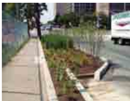
Curb extension with a planted swale that captures stormwater from the gutter: Beach 19th Street, Queens
