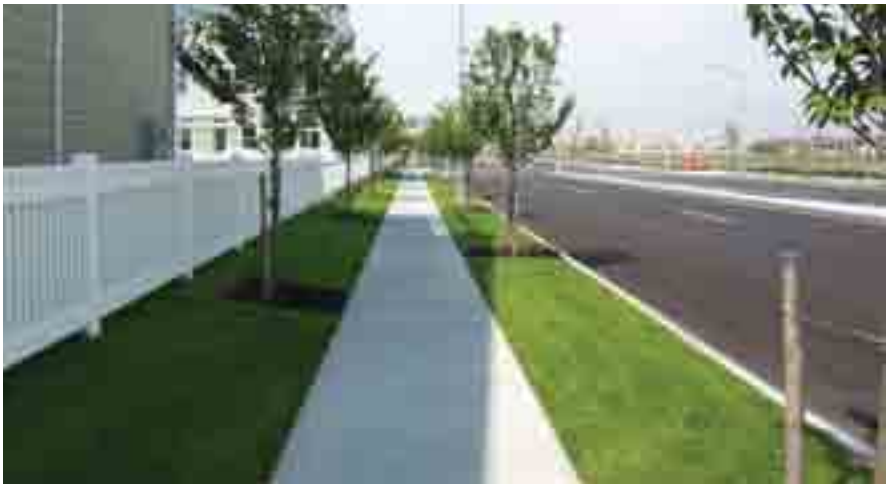
Concrete ribbon sidewalk: Rockaway Beach Boulevard, Queens
