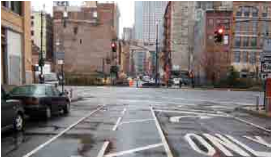
Median barrier: Canal Street, Manhattan
