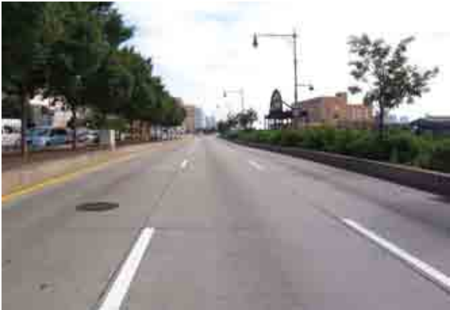
Typical concrete roadbed: West Side Highway, Manhattan
