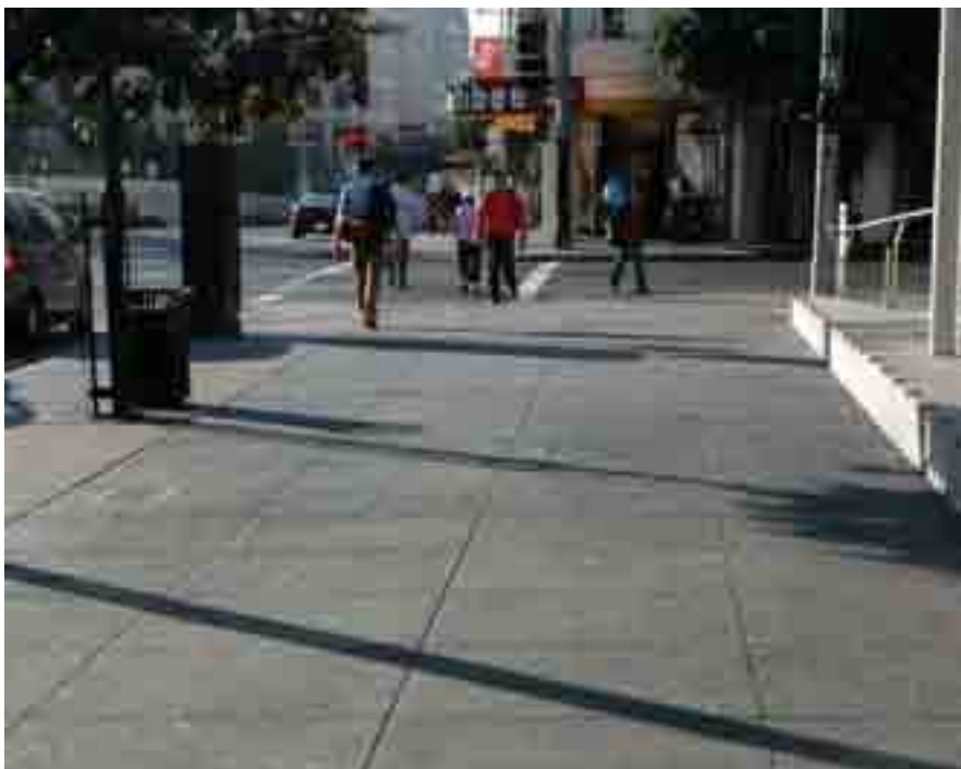
Tinted concrete sidewalk with silicon carbide treatment, shown with non-standard flag size: San Francisco, CA (Credit: Flickr user "Caribb")
