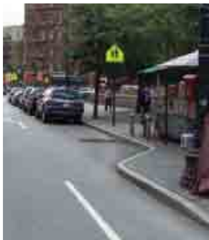
Curb Extension: Seventh Avenue, Manhattan
