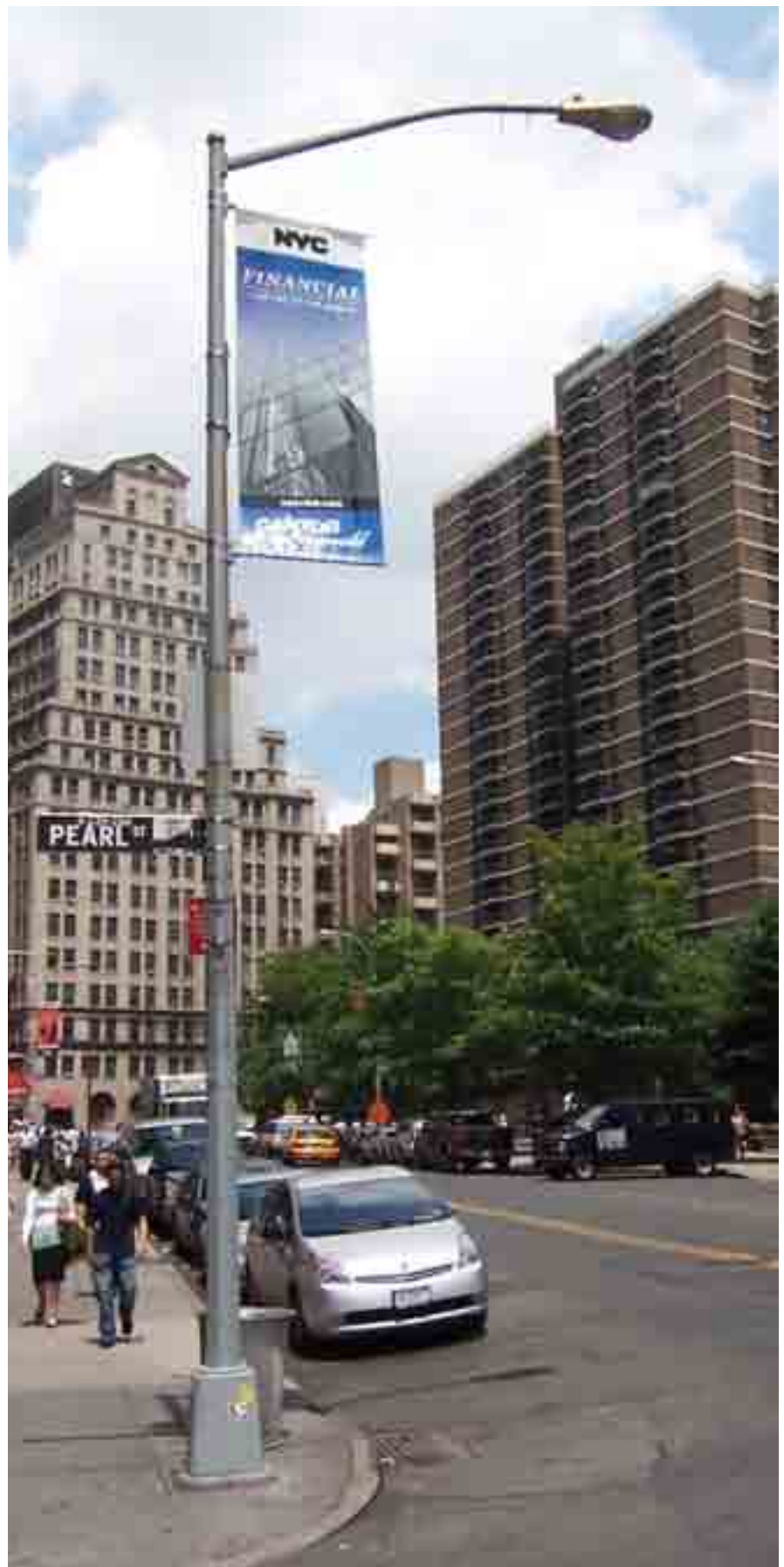
Cobra Head luminaire and octagonal pole: Pearl Street, Manhattan
