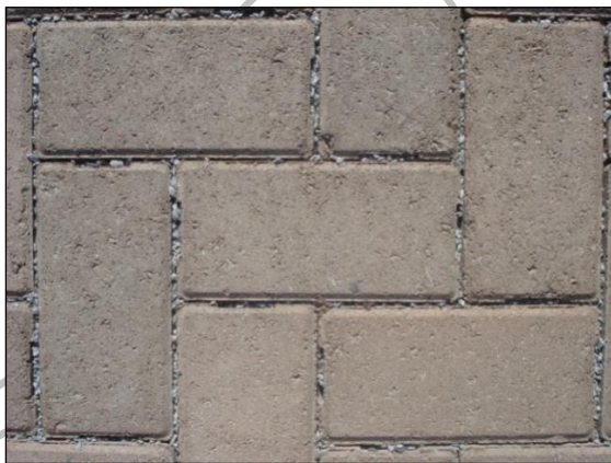
Figure 3.6: Permeable concrete block pavers with open joints and slotted ends filled with pea-sized gravel
