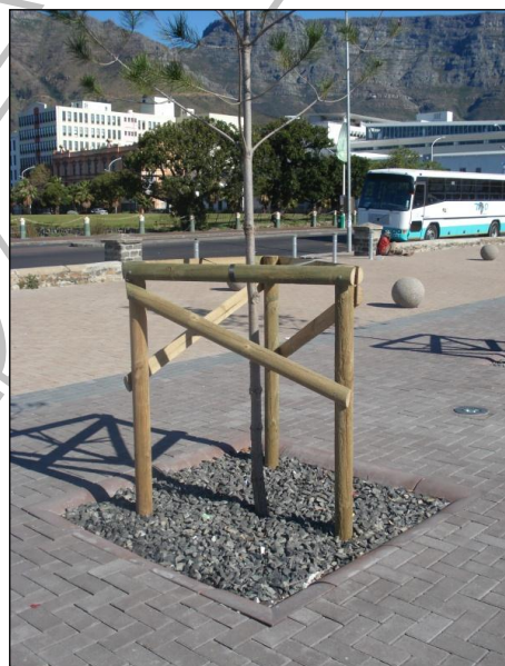
Figure 4.6: Bio-retention rut filled with a coarse aggregate and planted with a tree, Grand Parade, Cape Town
