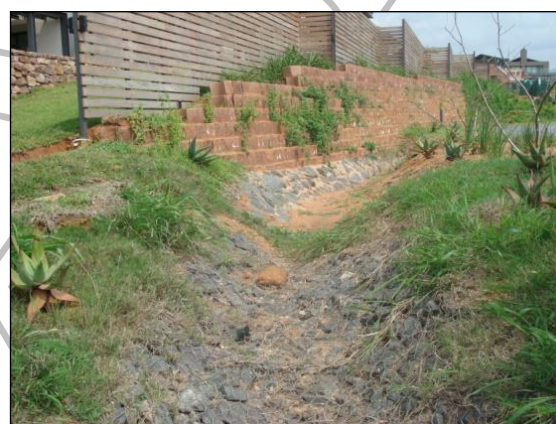
Figure 4.4: Gabion-lined dry swale, Hawaan Estate, Umhlanga
