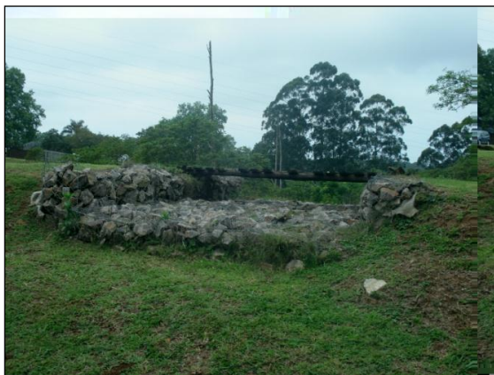
Figure 5.2: Detention pond emergency overflow structure, New Heritage Market, Hillcrest
