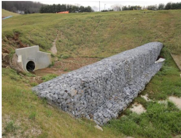
Figure 7.31-2C Forebay with Porous Berm (Gabion Rock)
