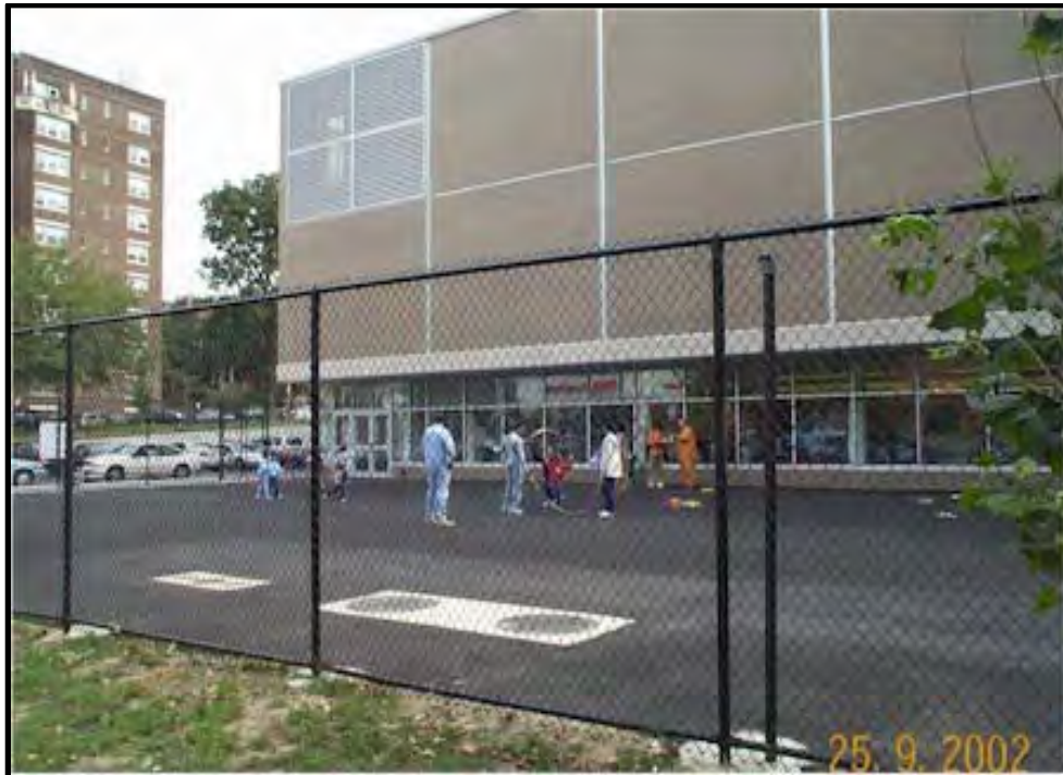
Photo 5-12. Porous Asphalt in Playground
