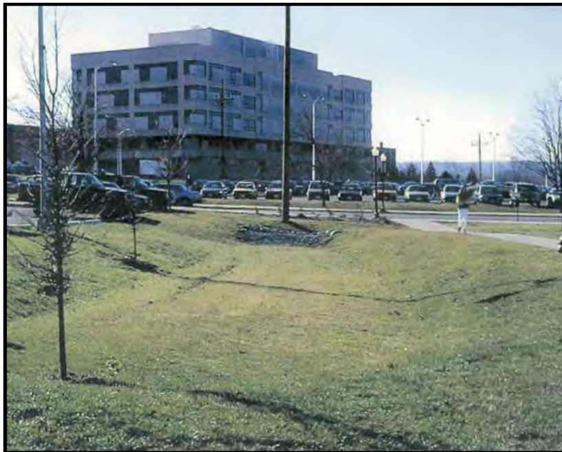
Photo 5-8. Vegetated Swale in a Commercial Setting
