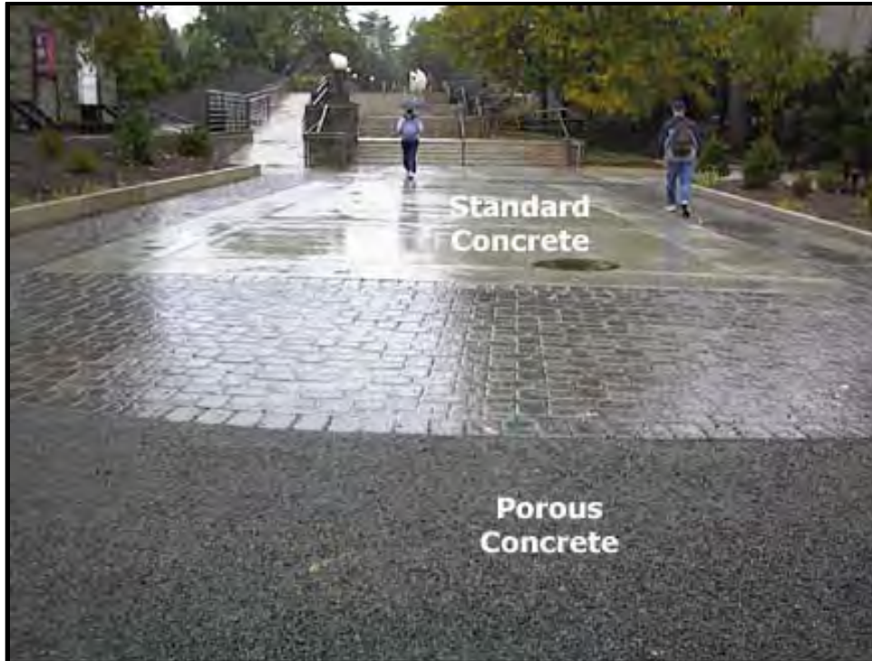
Photo 5-13. Standard and Porous Concrete
