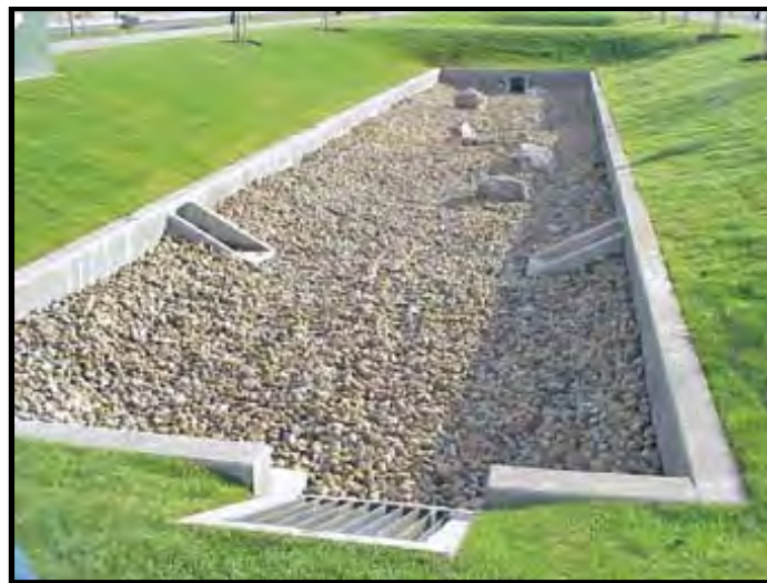
Photo 2-30. Surface Sand Filter (Source: City of Portland, OR)
