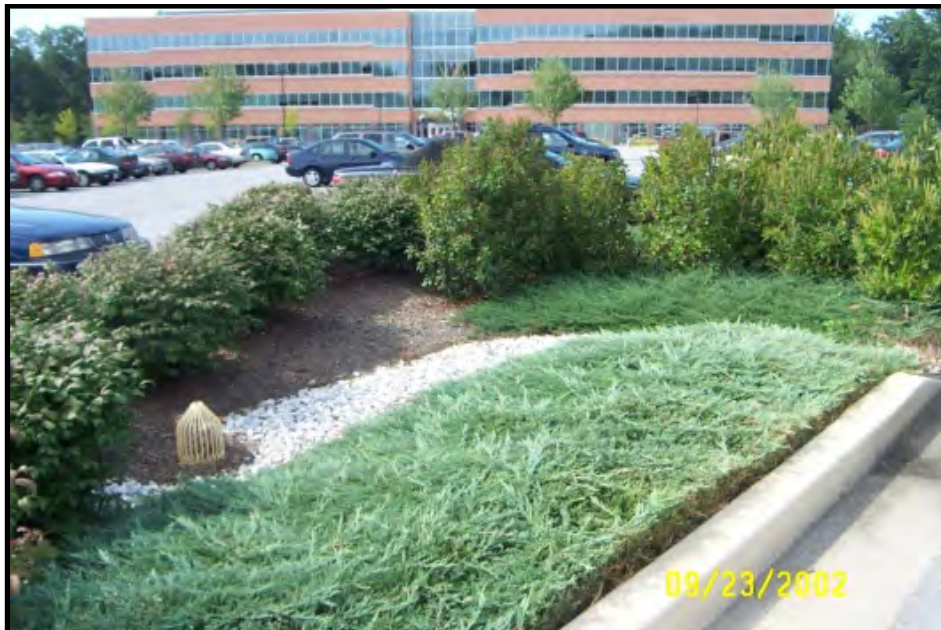
Photo 5-4. Inflow Entrance – Stone Channel
