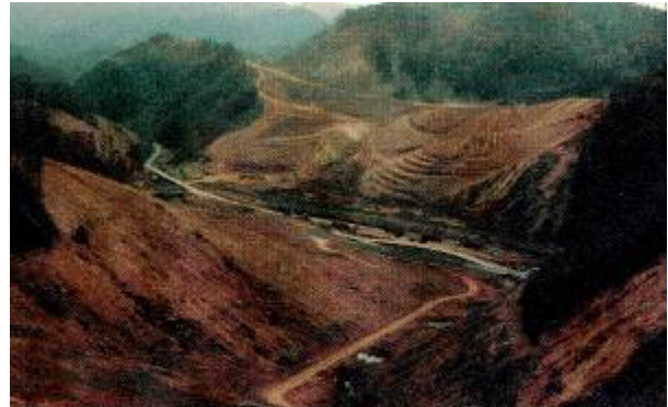
Terraces can be incorporated into the grading plan to shorten the length of the slope and to reduce the velocity of storm water flows (Source: Boaze et. al, 2000)
