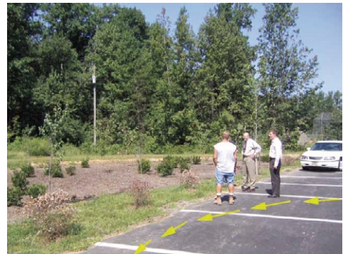
Some site runoff by-passes bioretention because of inadequate slope of filter strip.
