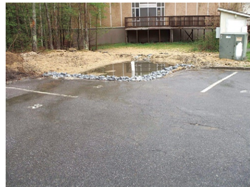
New BMP retrofit after first storm.
