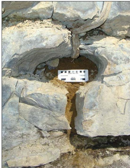
Figure 13. Dissolution opening in exposure of Catheys Formation, Center Hill Dam
