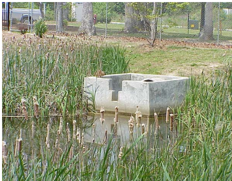
Enhanced Extended Detention Basin – Shallow Marsh. Note multi-stage weir principal spillway and deep water pool (18" – 48" depth).
