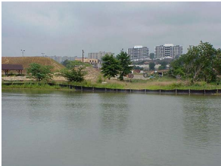
Retention basin in ultra-urban setting (under construction).
