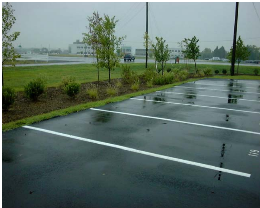
Bioretention Basins in office setting parking lot.
