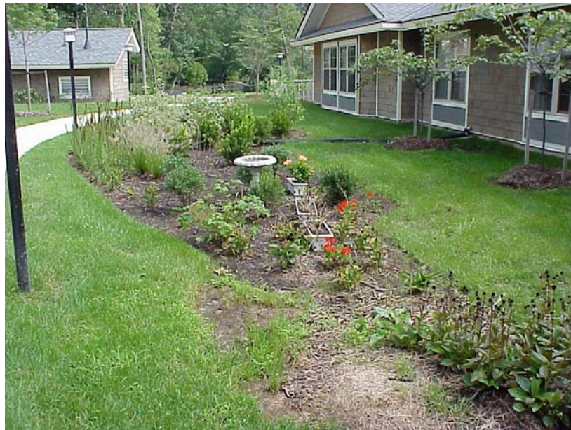
Bioretention Filter in multi-family residential setting.
