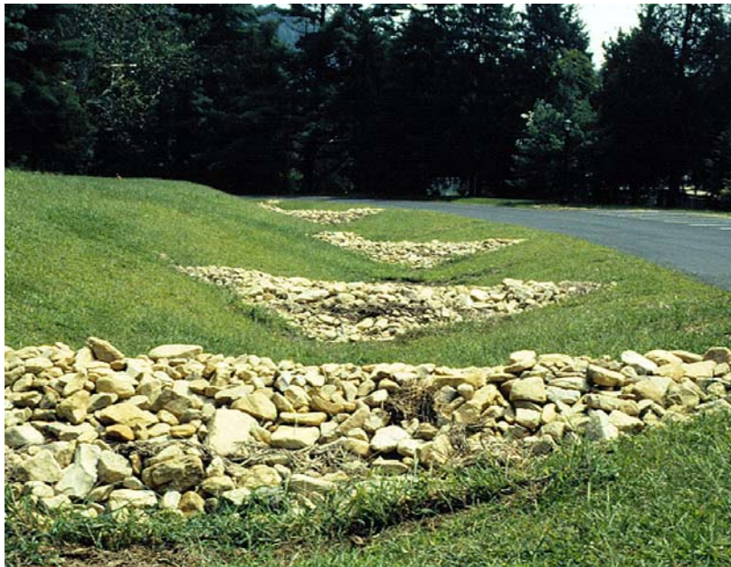
Grass Swale with Check Dams. Note significant channel storage capacity created by check dams. Notched center allows safe overflow without scour around sides.
