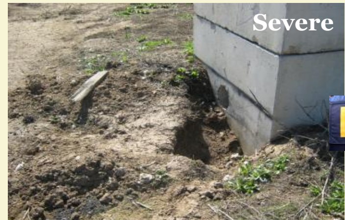
Check underdrain or outfalls for evidence of media migration
